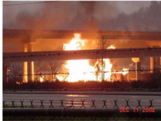
Photo 1. Puyallup River Bridge Railroad Tanker Fire
