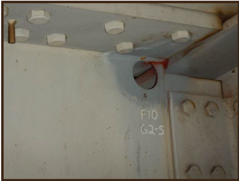
Crack Arrest Hole
