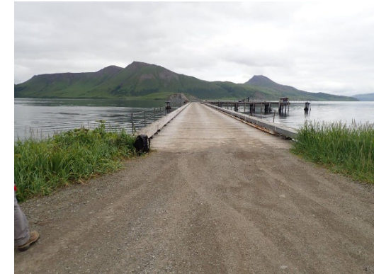
False Pass City Dock
