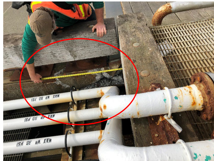
New Dock / Old Dock Joint (RT)
