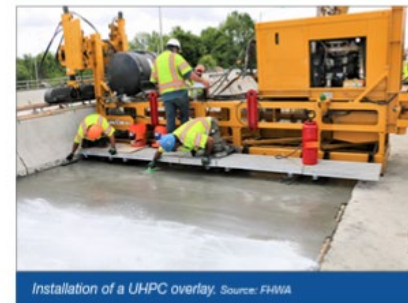
Installation of a UHPC overlay. Source: FHWA
