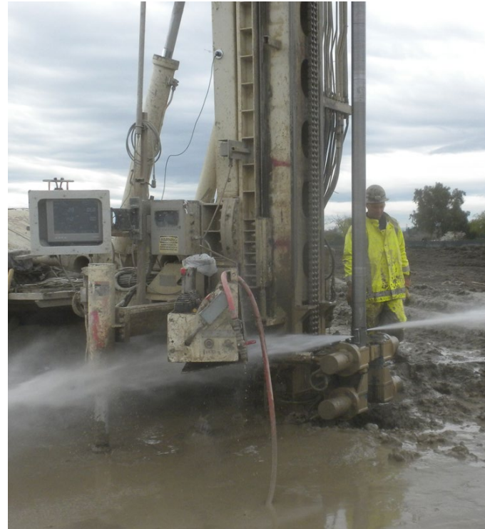
Jet Grouting BART Warm Springs Extension Project
