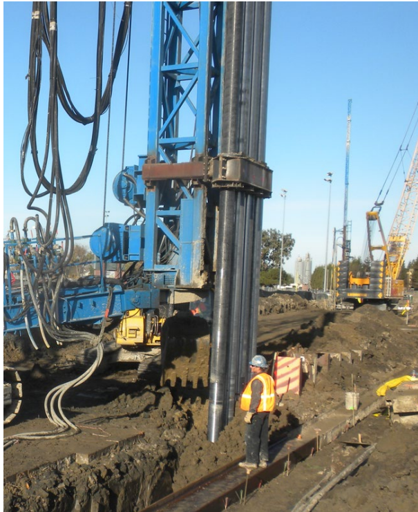
Deep Soil Mixing BART Warm Springs Extension Project
