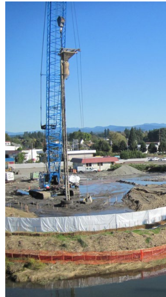
Stone Columns WSDOT Ebey Slough Bridge Project
