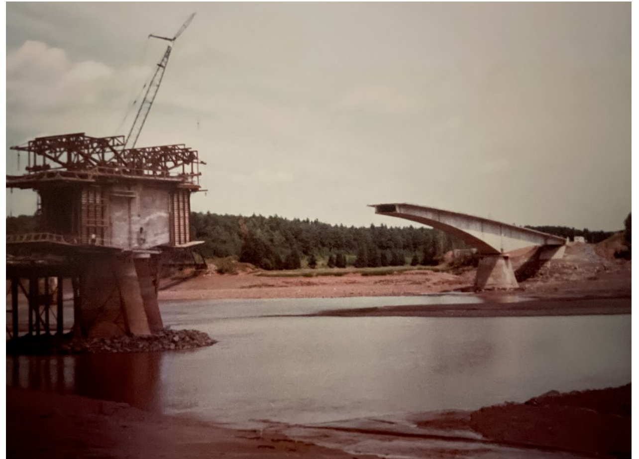
West Span – Summer construction
