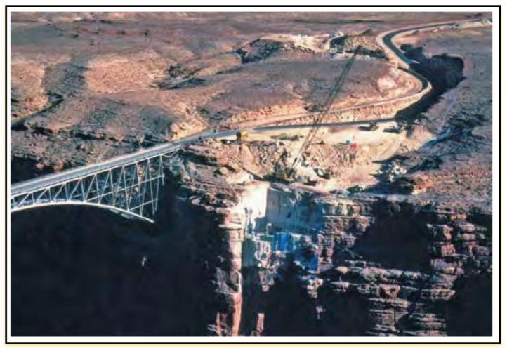
Using cantilever erection method to erect steel over canyon.
