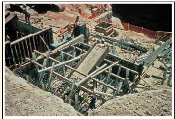
The top chord of the steel truss was anchored to a tieback footing by steel cables embedded into the rock.
