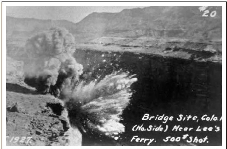
Dynamite was used to blast notches into the canyon walls in order to anchor the bridge into solid rock. Since there were no environmental requirements, the excavated rock was allowed to fall into the Colorado River. Photo courtesy of ADOT.
