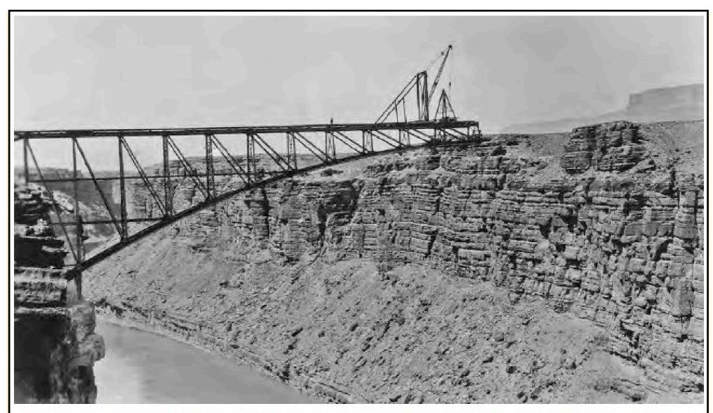
The Flagstaff half bridge cantilevering out 308' over the Colorado River as construction on the other half bridge begins on the Fredonia side of the river. Photo courtesy of ADOT.
