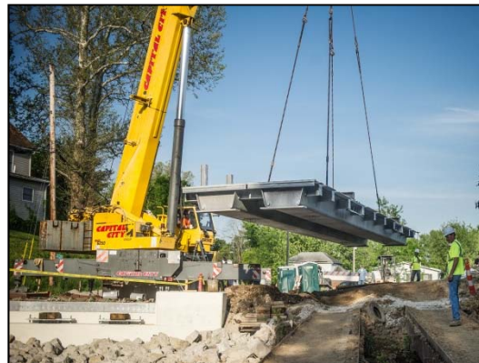
Integrated Deck-to-Tub Girder
