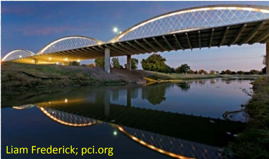
West 7 th Street Bridge – Ft. Worth, TX (2011)
