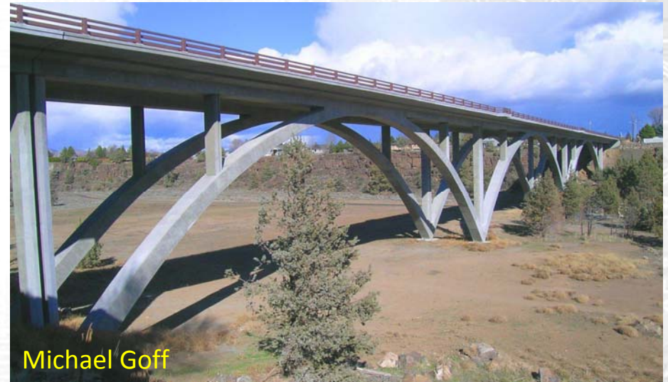
Maple Avenue Bridge – Redmond, OR (2006)
