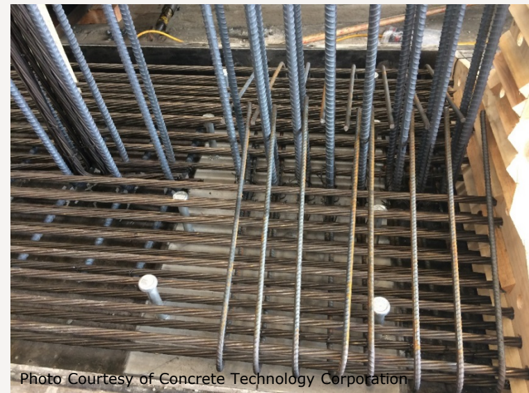
EMBEDDED GIRDER PLATE
