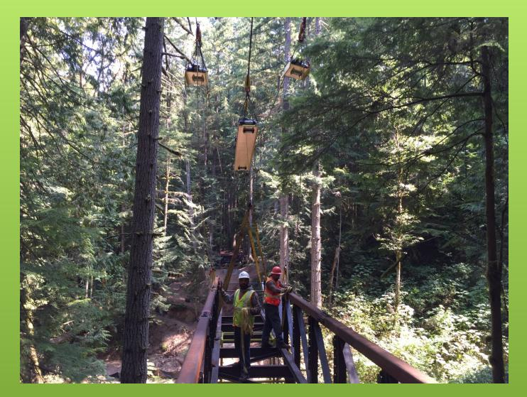
Remote control, 12V battery operated travelers.
