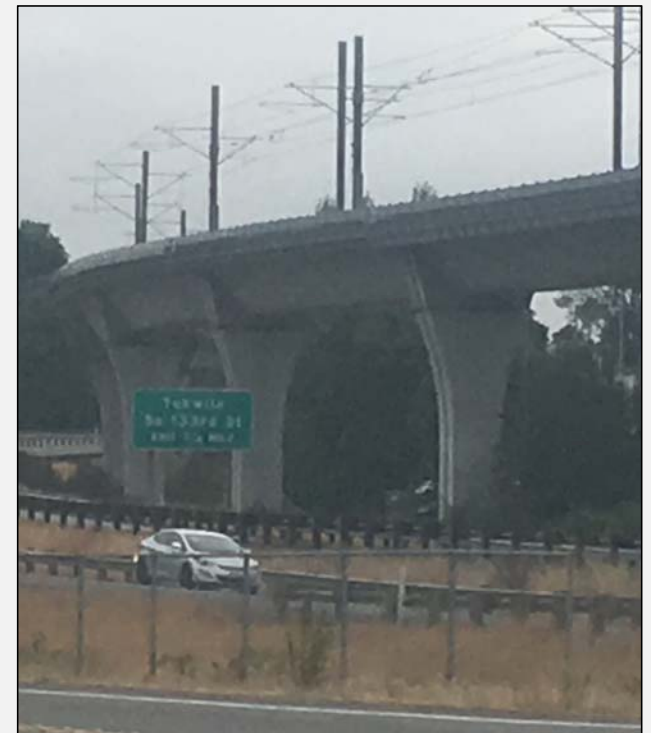
Central Link: Seattle to SeaTac Aerial Guideway: 4.2 miles
