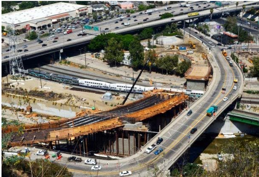
Stage One Under Construction
