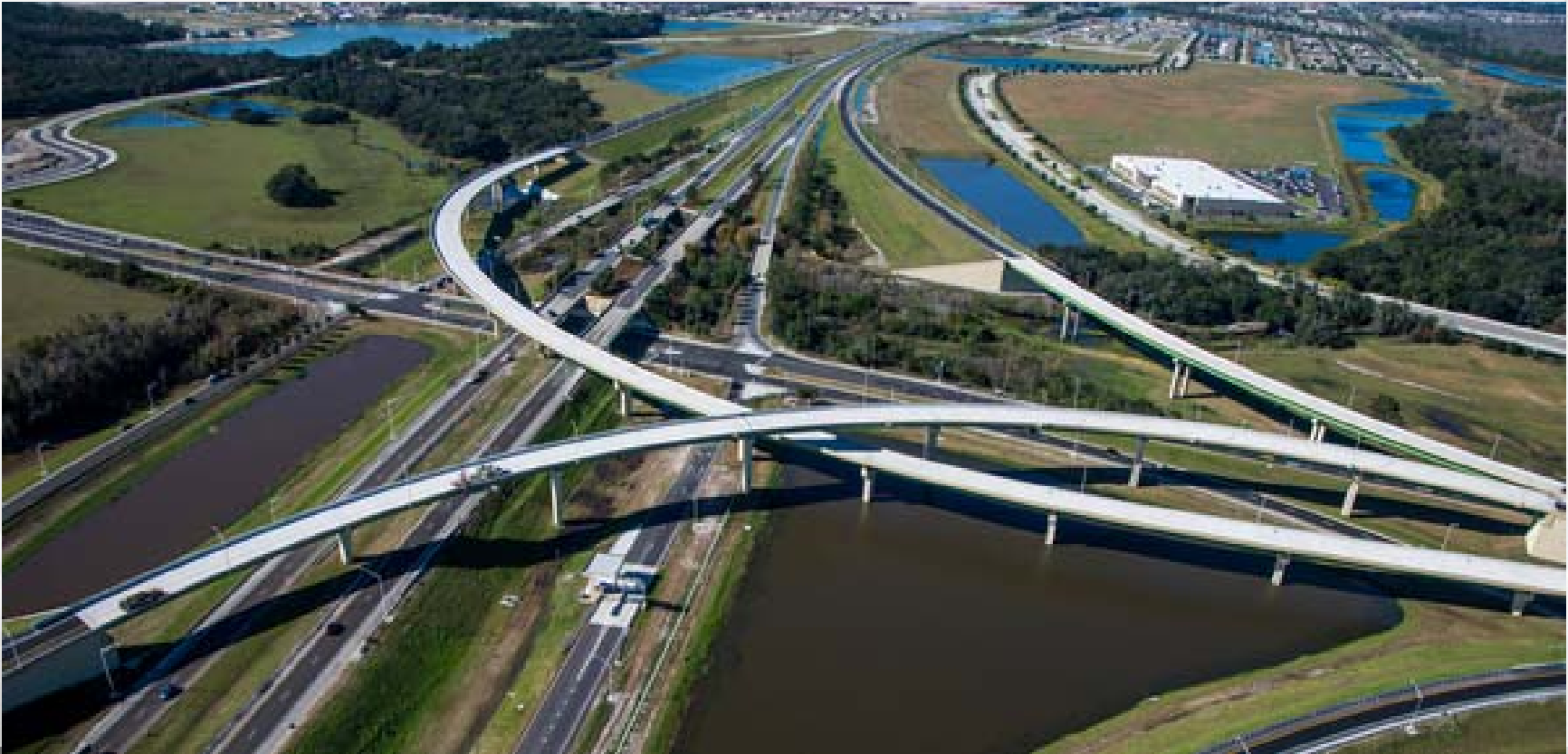
Boggy Creek Interchange – Orlando Florida
