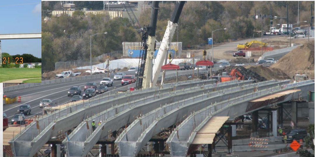
Long Span Spliced Girder Bridges using Standard Bulb Tee Sections
