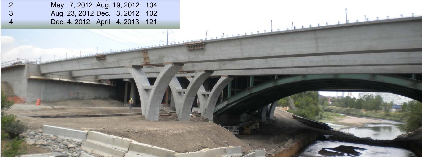
Precast Piers and Full Depth Precast Deck
