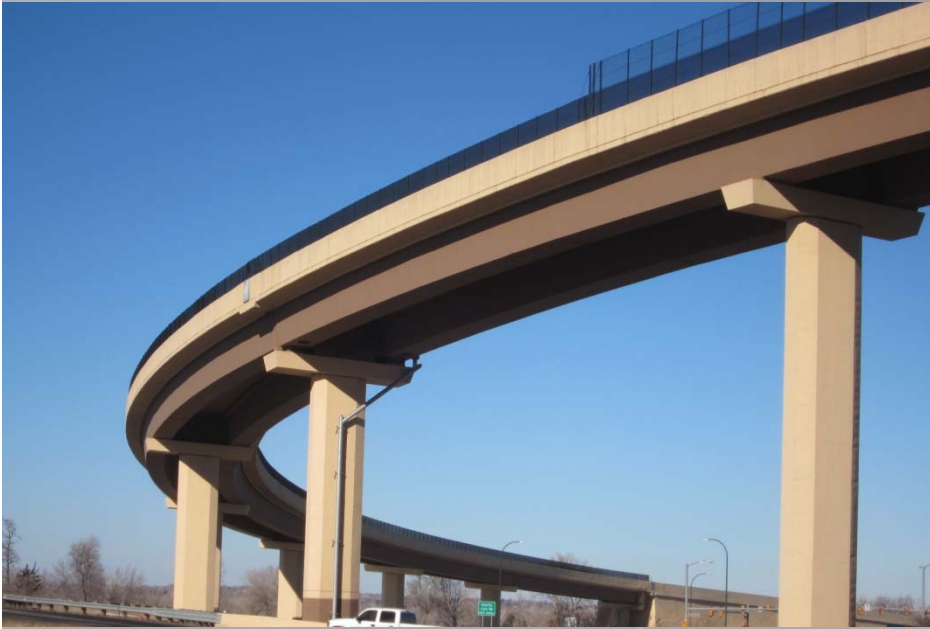
IH25 SB Ramp K, Denver CO
