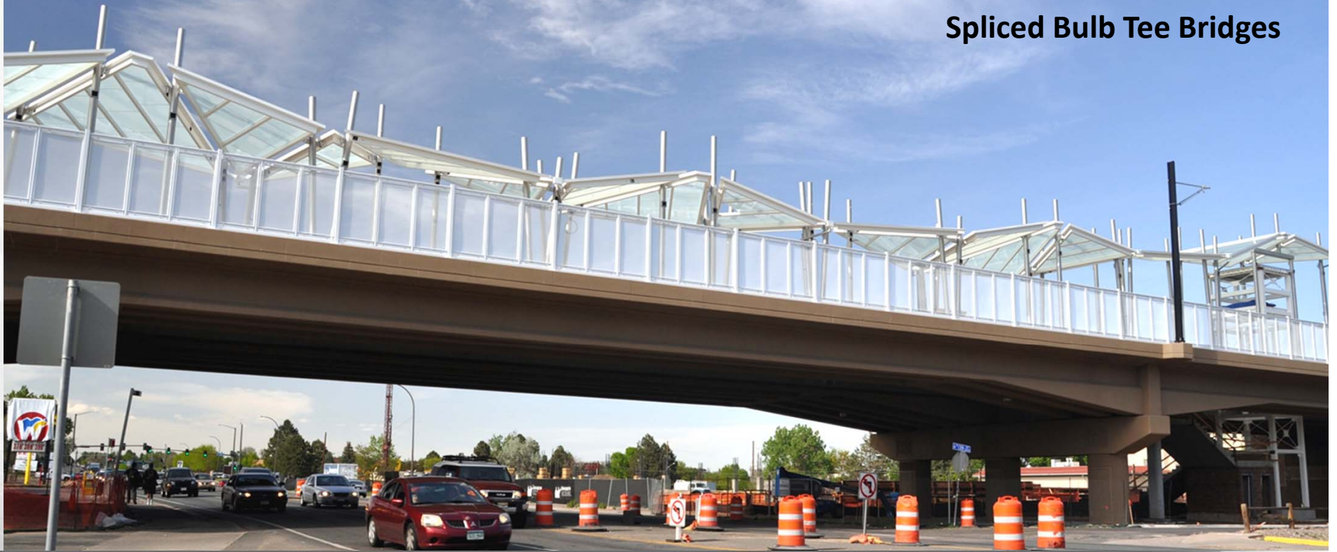
Wadsworth Light Rail Bridge and Station, Denver Colorado
