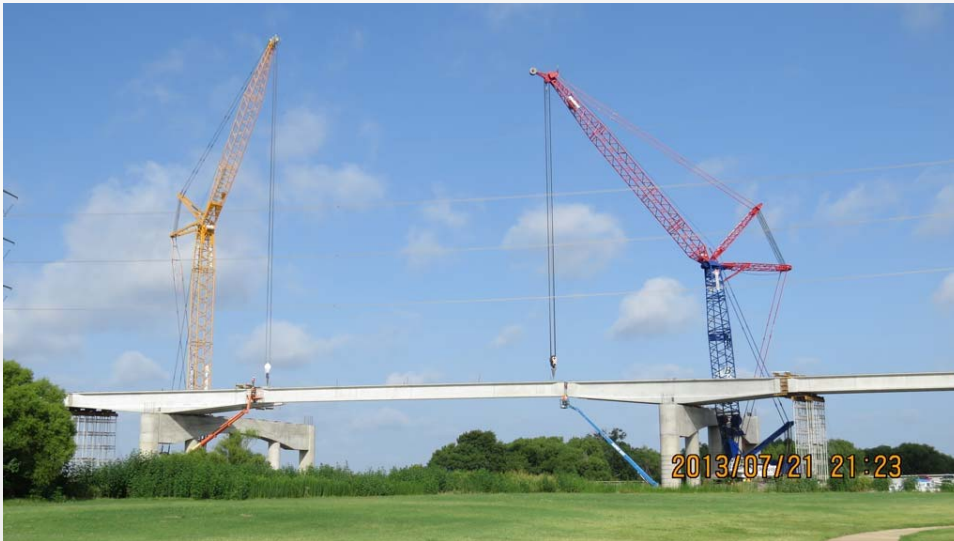
Long Span Spliced Girder Bridges using Standard Bulb Tee Sections
