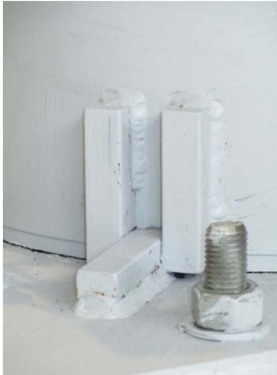
Shear key to restraint twist
