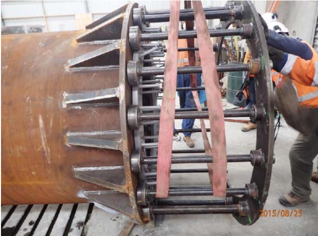
Construction photos, courtesy of Routledge and Cowan (2016)
