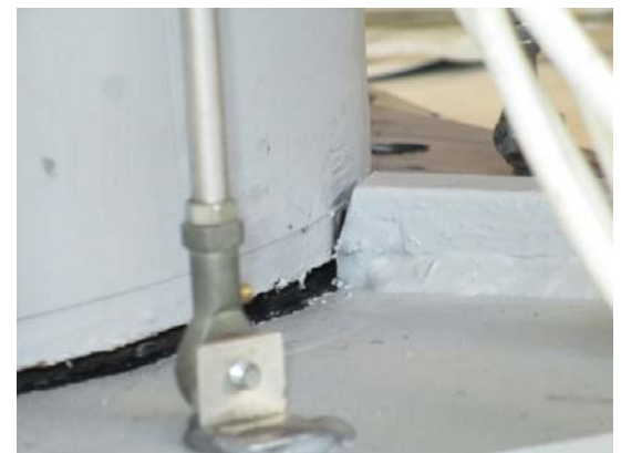
Typical rocking joint in the bent
