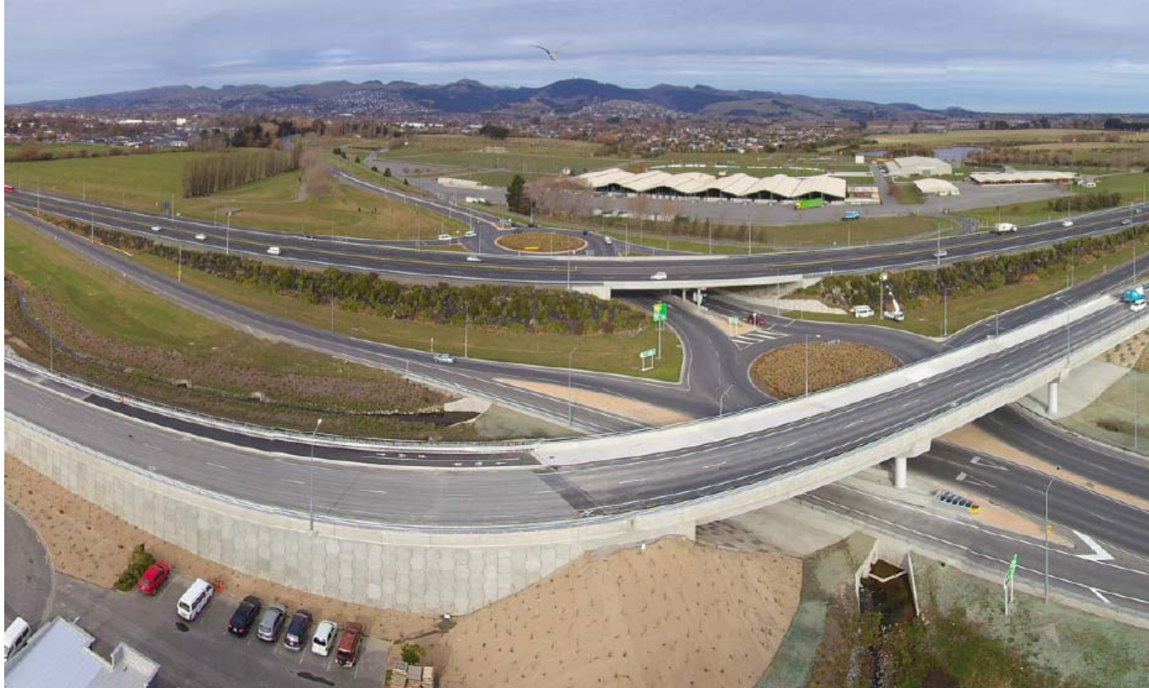
Completed Bridge, courtesy of Hawkins (2016)
