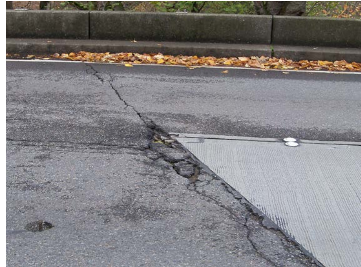
Joints in Pavement
