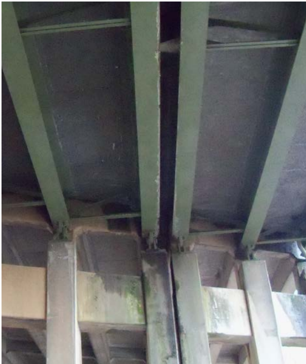
Corroded Steel Girders
