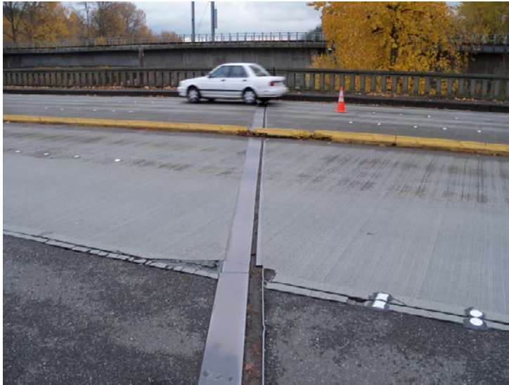
Expansion Joints – Transverse & Long.
