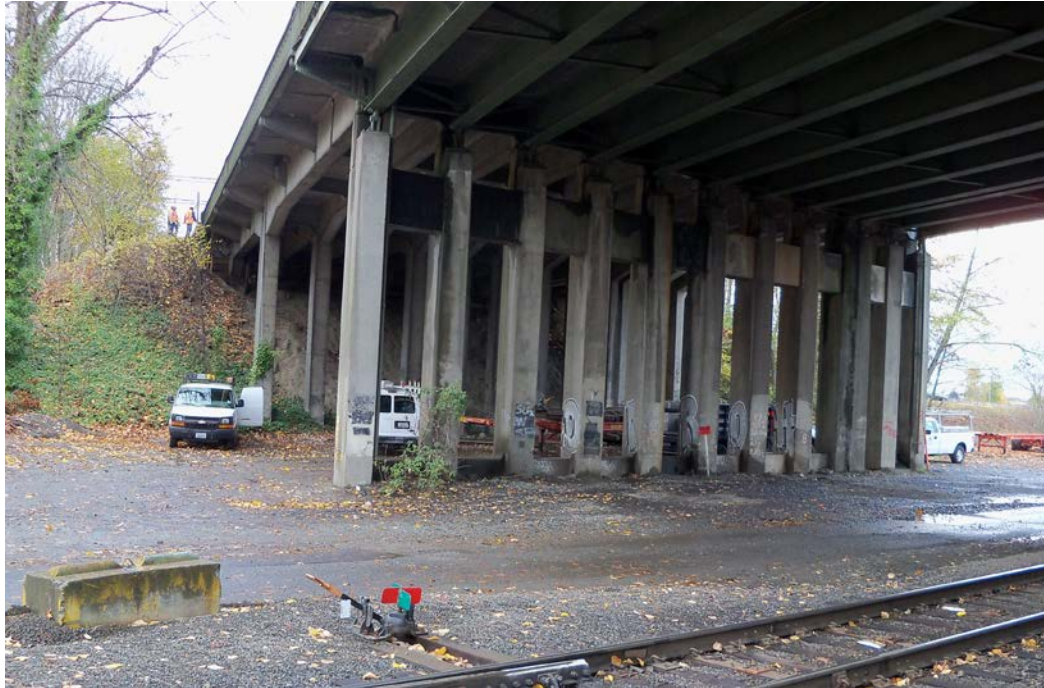
Steep slope with Liquefiable Soils near Pier 5
