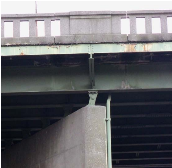
Wall Pier with Steel Bearing
