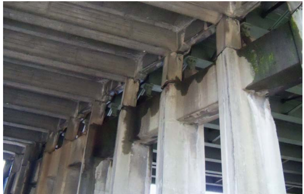
Concrete Spalls
