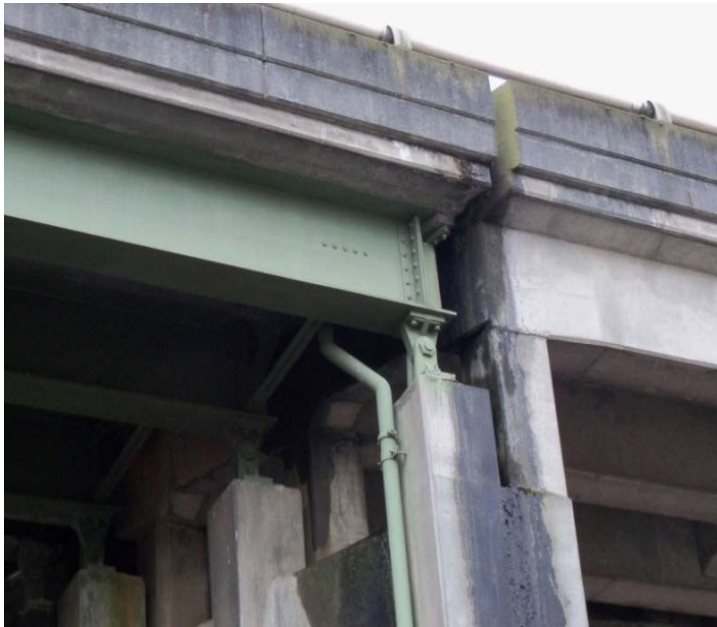
Transverse joint at Pier 4
