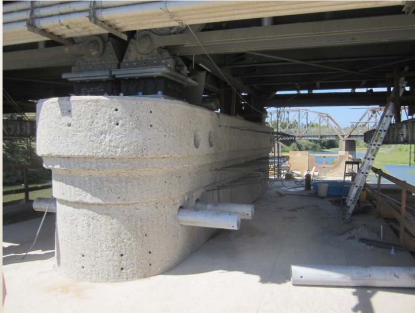
Pipe Dowels for Shear Transfer To New Cap Beam
