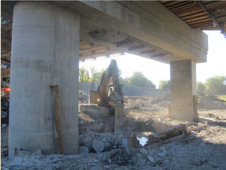
Self Supporting Cap Prior to Infill Wall Construction
