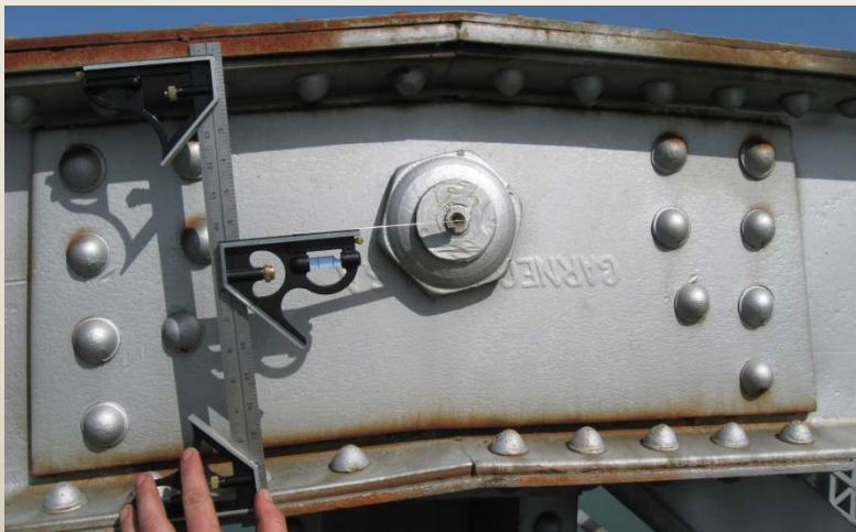
Always Check Truss Pin Eccentricity
