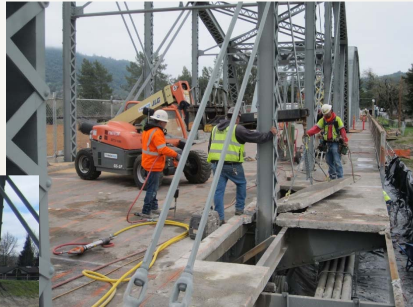
Staged Deck Removal
