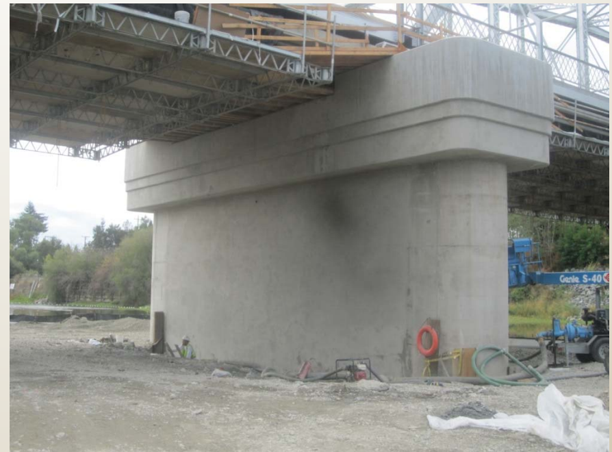
Completed Super Bent
