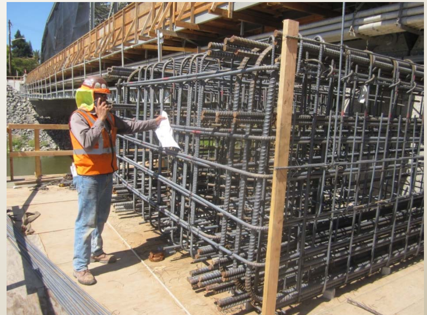
Pipe Dowels for Shear Transfer To New Cap Beam
