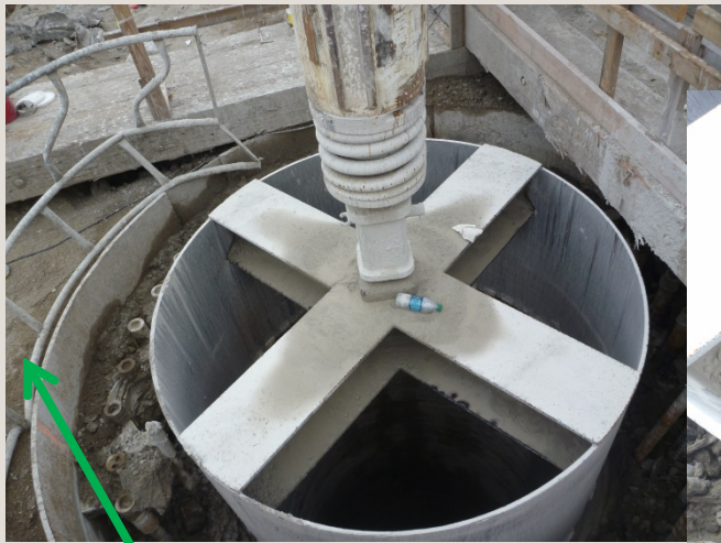
Existing shaft casing
