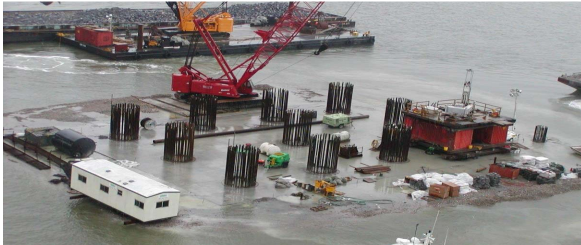
West Tower Drilled Shaft Foundations Arthur Ravenel Jr. Bridge, Charleston SC
