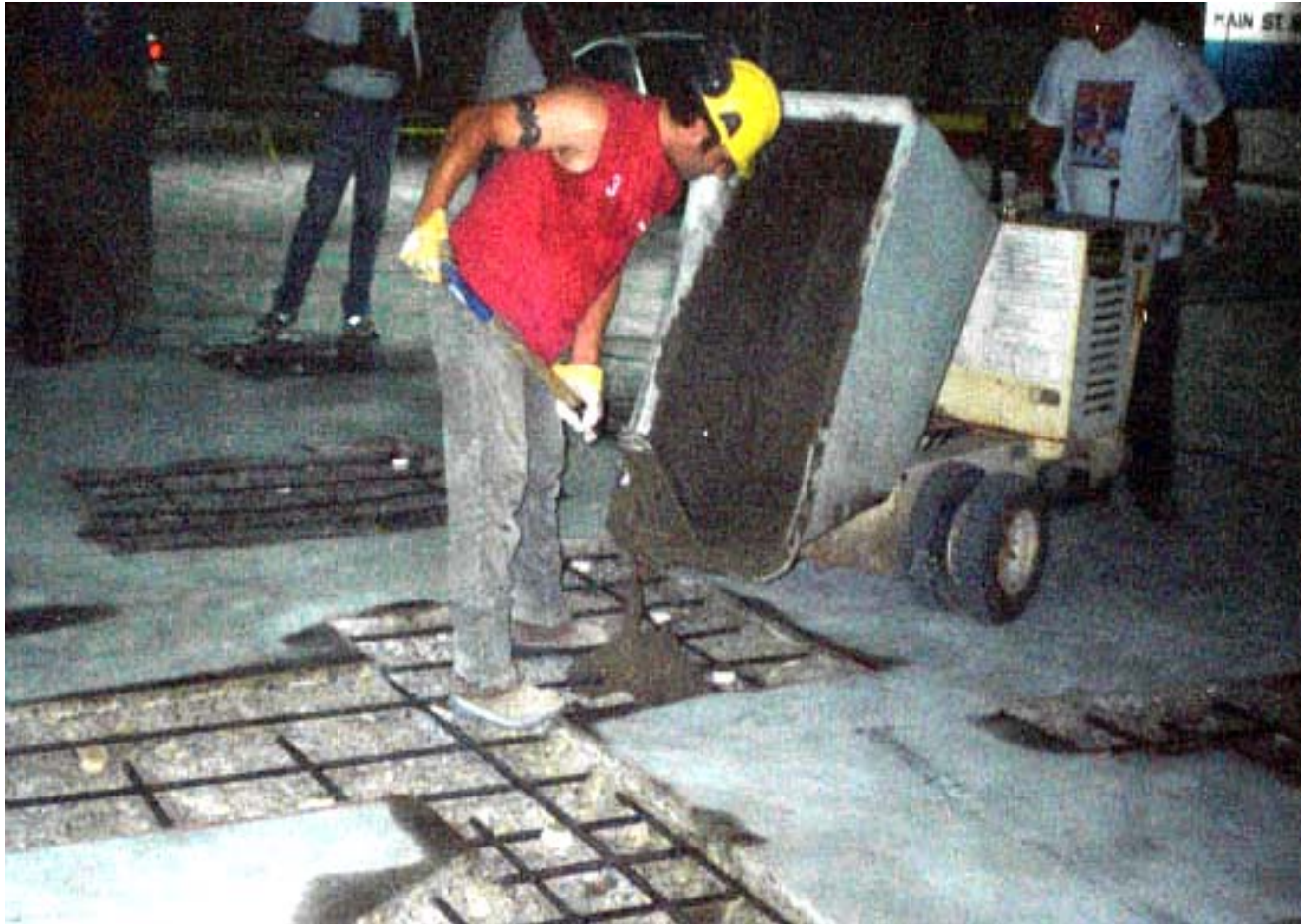
Embedding anodes with repair material.
