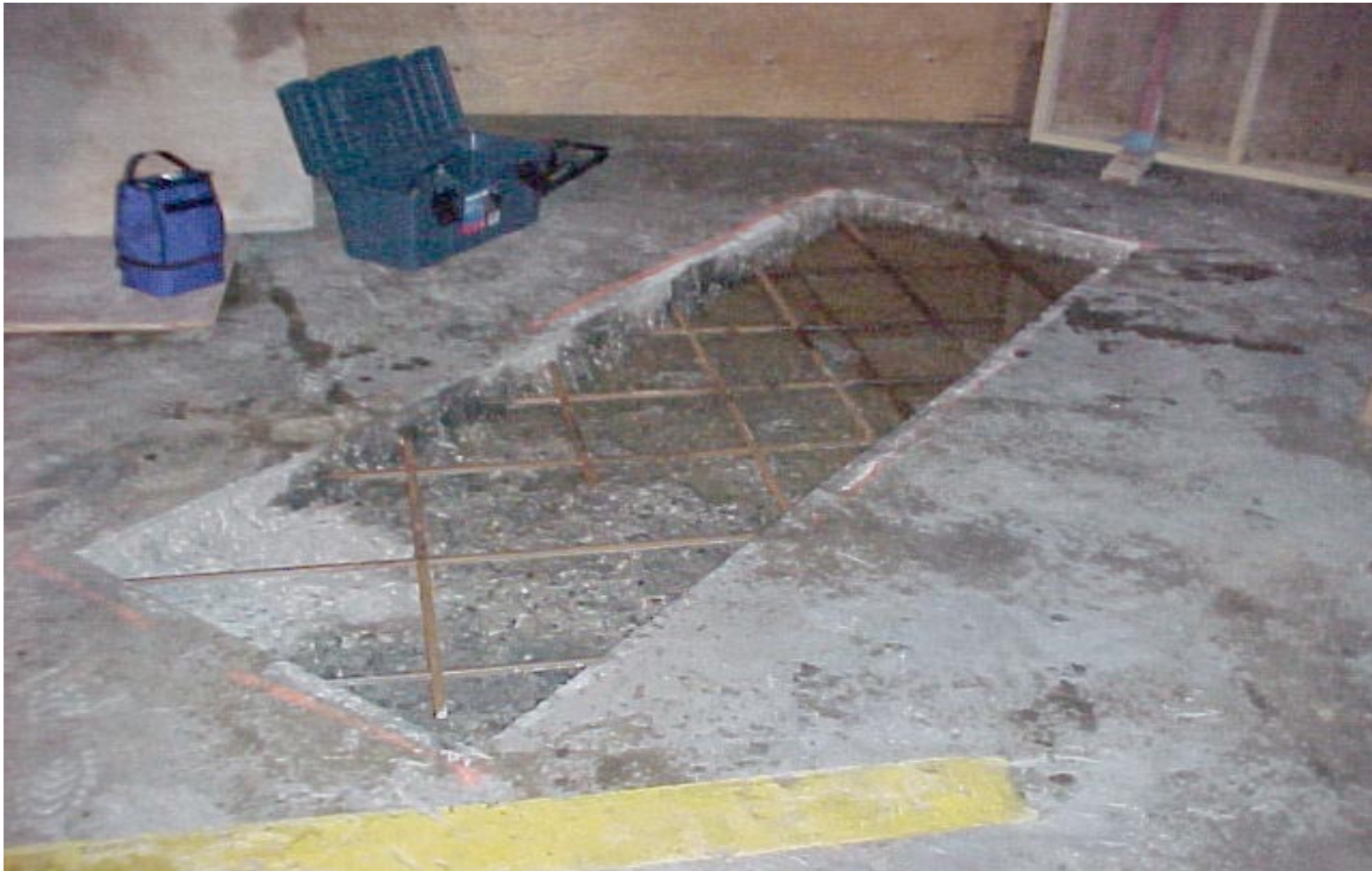
Saw cut and cleaned repair area.
