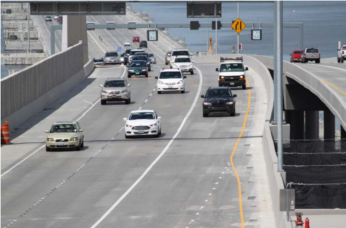
Open to Traffic on April 11, 2012, looking west from Medina.
