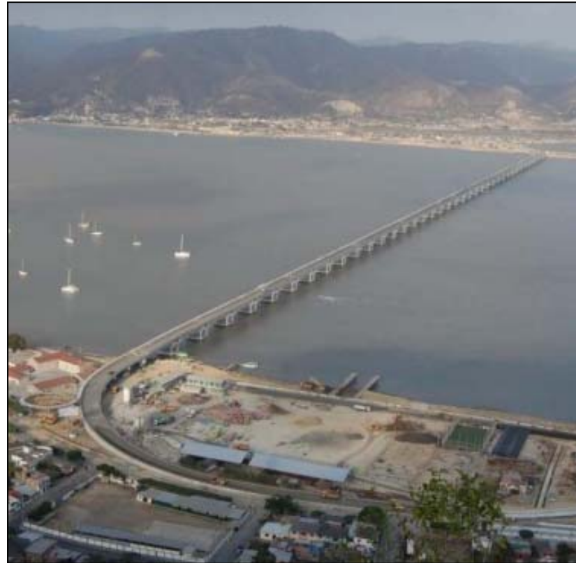
The 6500 ft long isolated Los Caras Bridge in Ecuador was open to traffic immediately after the nearby 7.8 Magnitude Earthquake struck in 2016.
