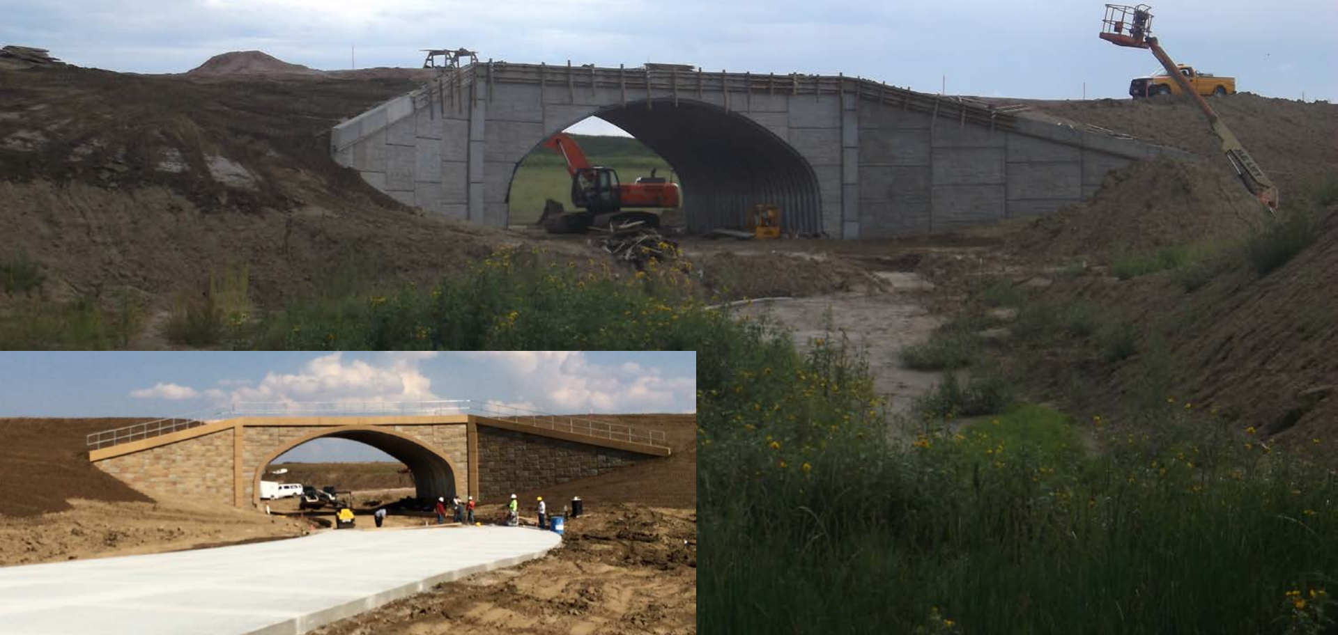
Randolph, Nebraska E-80 Cooper Engine, 3.67 ft cover, ~50 ft span
