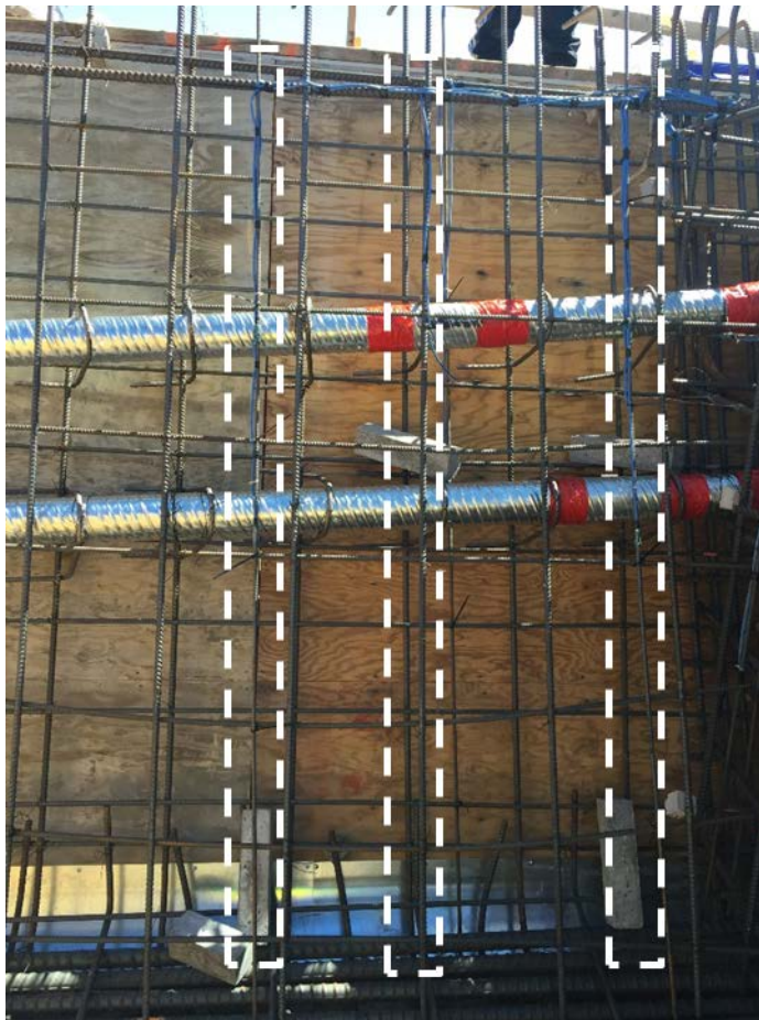
Installed sister bars in the external web
