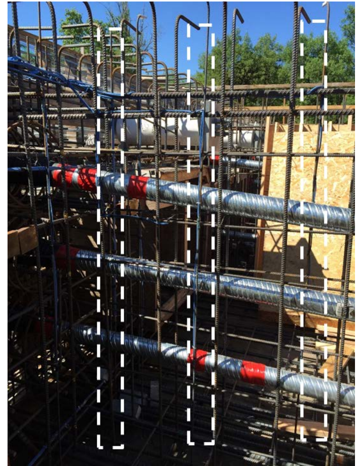
Installed sister bars in the internal web
