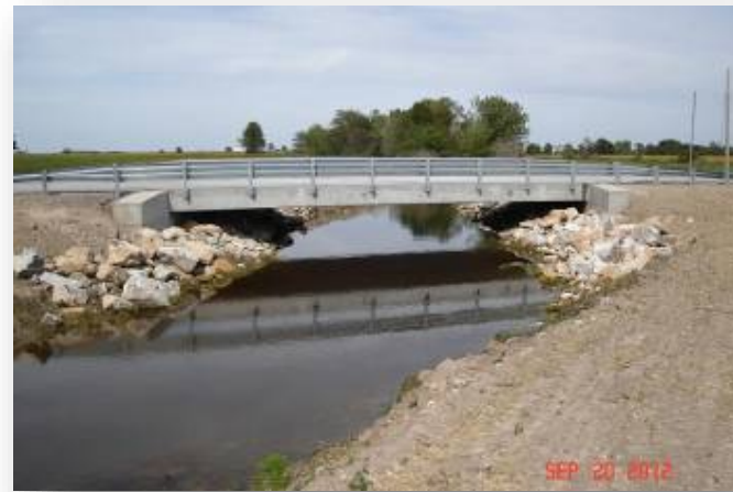
Audrain County, MO Bridge 336 Built 2012 Precast 6 Hollowcore Slab Girders 50.5 ft. Span 24 ft. Roadway Width 2 ft. Structural Depth 20° Skew
