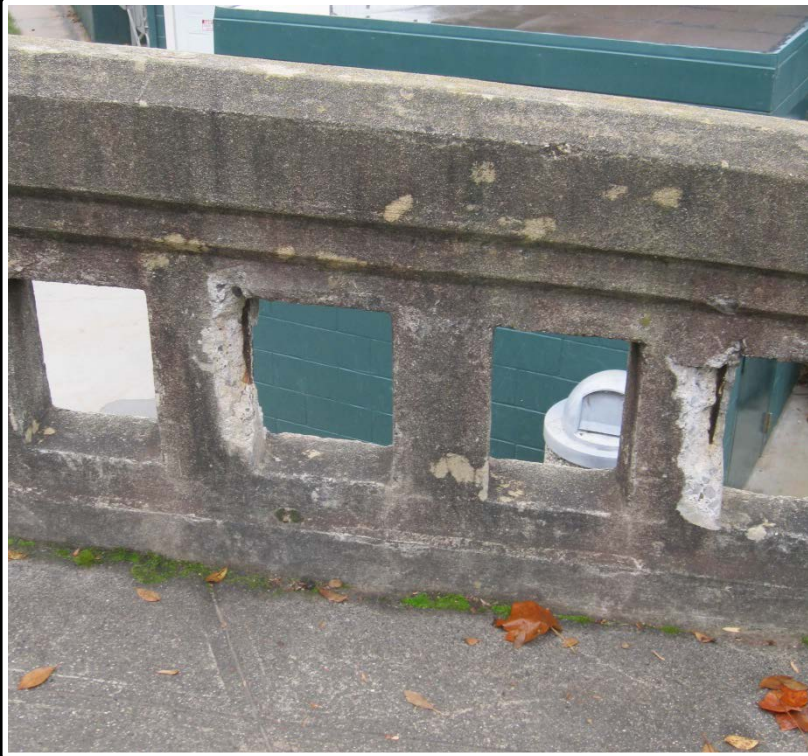
View the south railing
