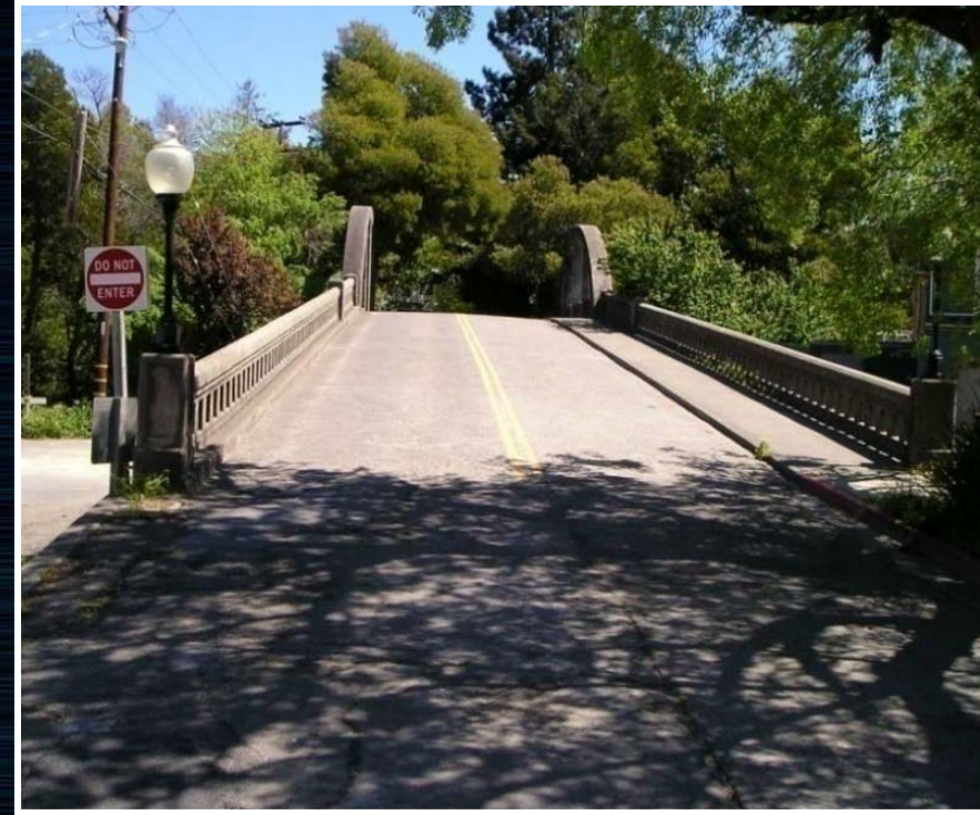
View of bridge approach deck taken from west side
