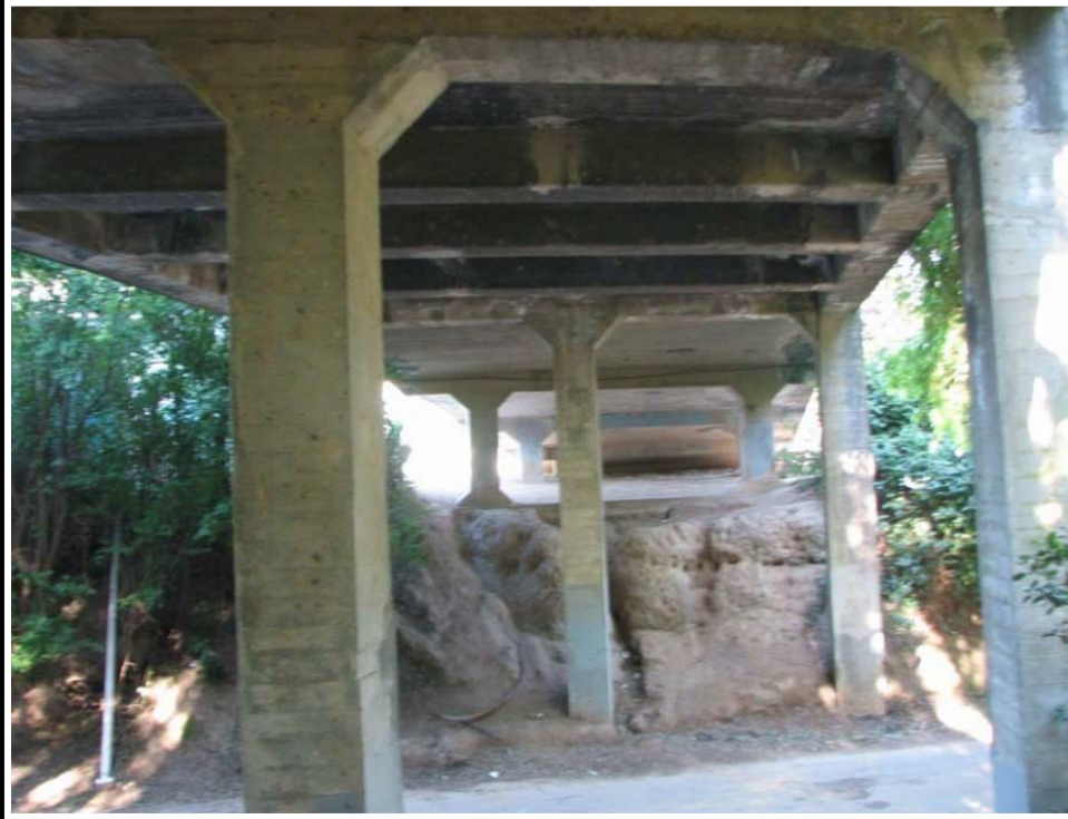
Underside of bridge taken from east side
