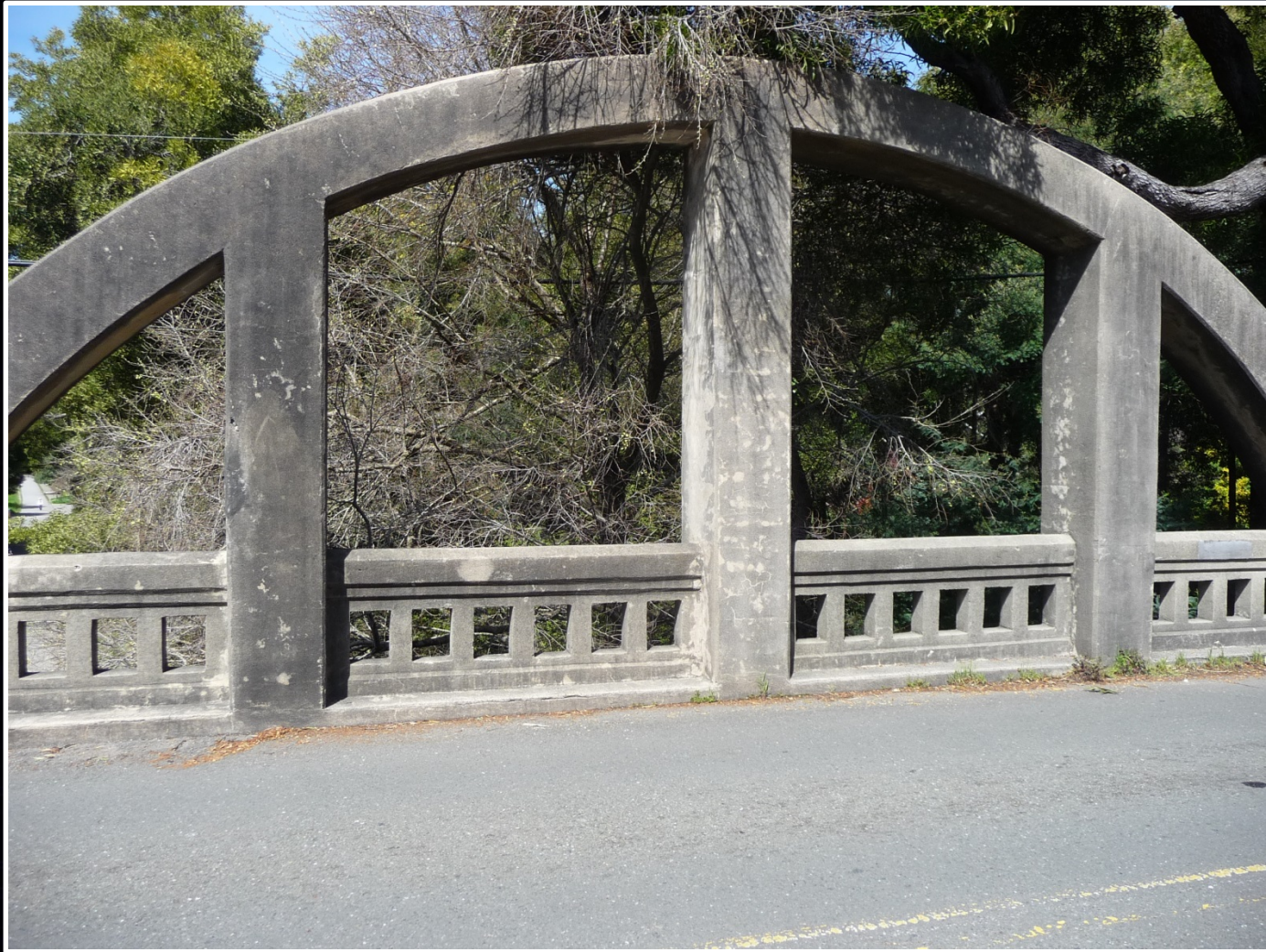
View of the south arch span taken from the westbound lane
