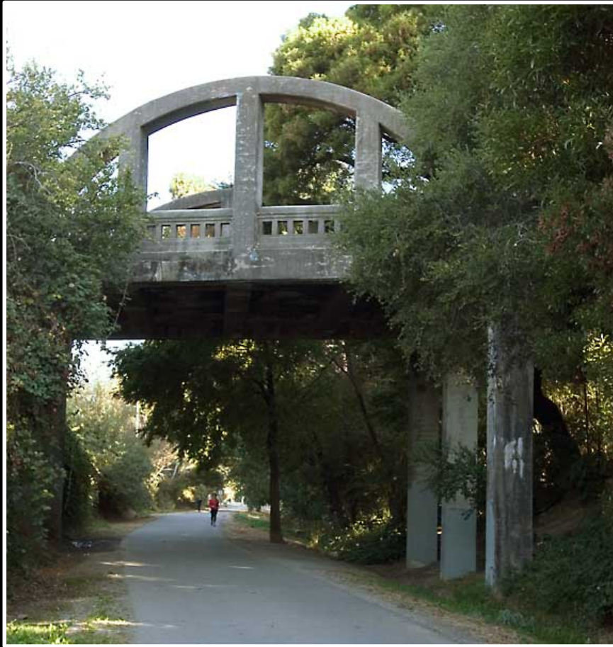
View of north side of arch span taken from bike path
