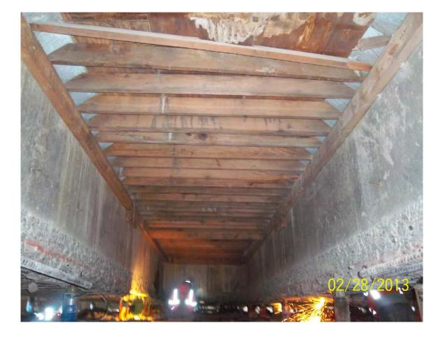
Existing top slab formwork was removed
