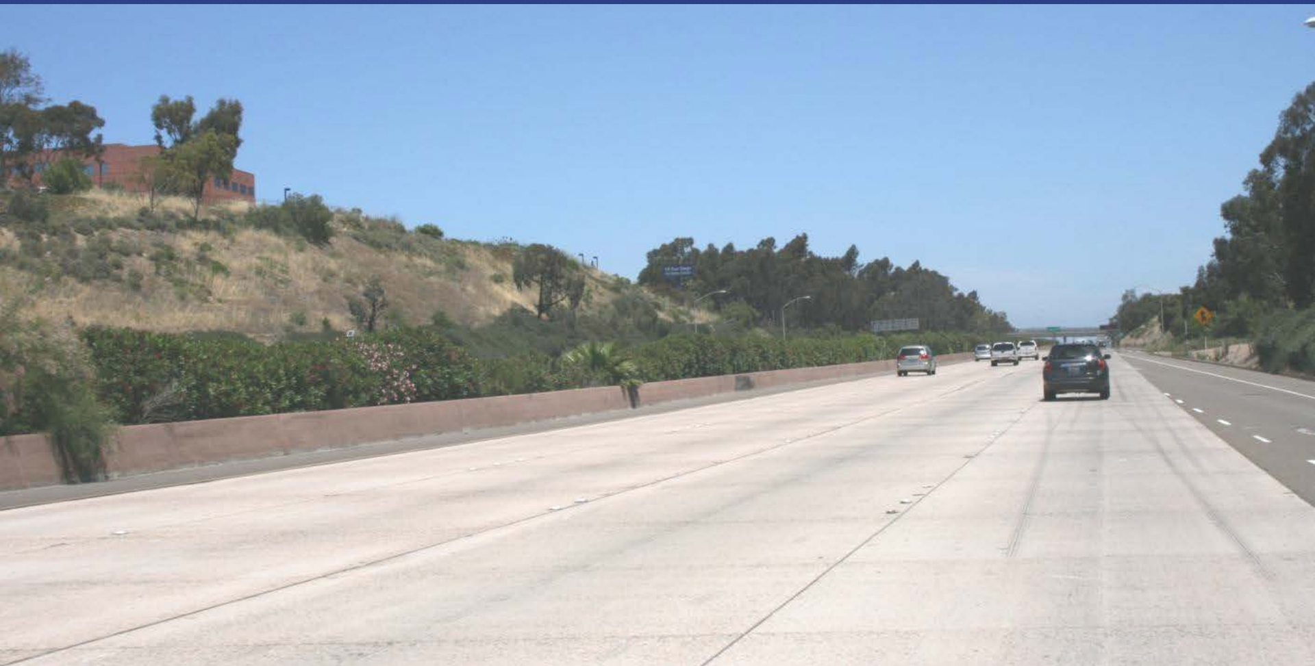
Existing Interstate 5 Northbound
