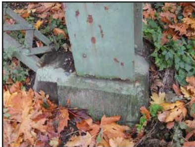
FOUNDATION P3a (6W)
