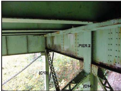
PIER 2 & 3 DIAGONAL BRACING LOOKING EAST
