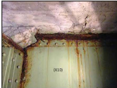
PIER 5 (B10) CROSS GIRDER (X10) TOP FLANGE
