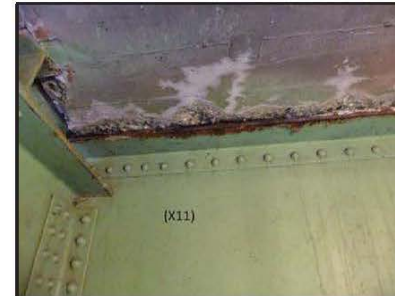
PIER 5 CROSS GIRDER (X11) TOP FLANGE
