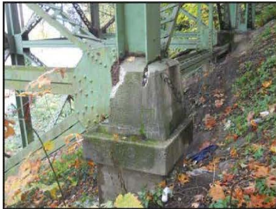
FOUNDATION P2a (6W)
