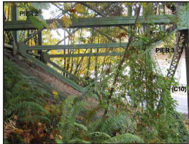
PIER 2 & 3 DIAGONAL BRACING LOOKING WEST
