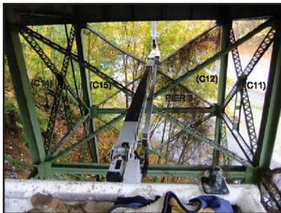
PIER 2 & 3 DIAGONAL BRACING LOOKING WEST
