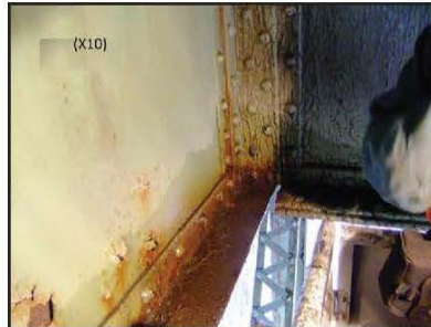
PIER 5 CROSS GIRDER (X10) BOTTOM FLANGE
