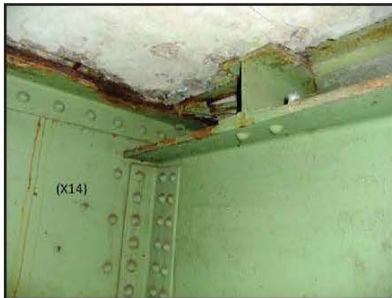
PIER 3 CROSS GIRDER (X14) TOP FLANGE
