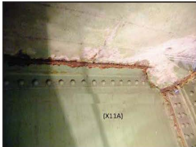
PIER 5 CROSS GIRDER (X11A) TOP FLANGE
