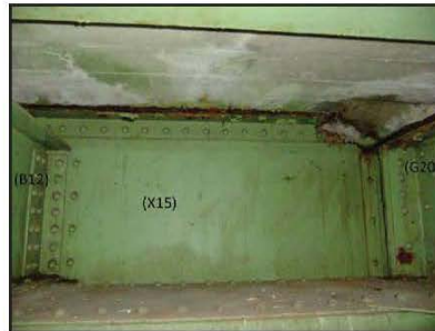
PIER 3 CROSS GIRDER (X15) TOP FLANGE
