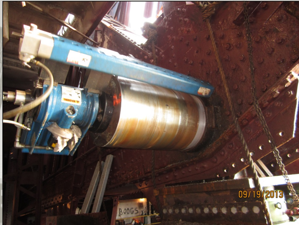
Field Machining - Grease grooves removed, rough cut complete
