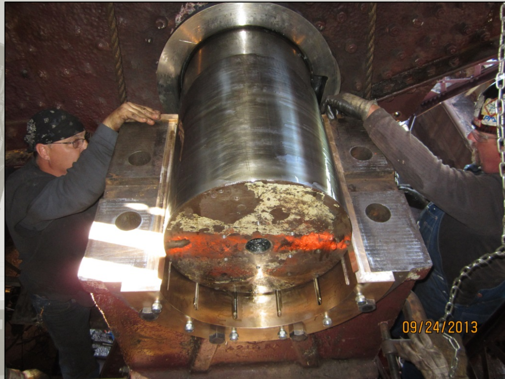
Trunnion bearing base and bushing at installation
