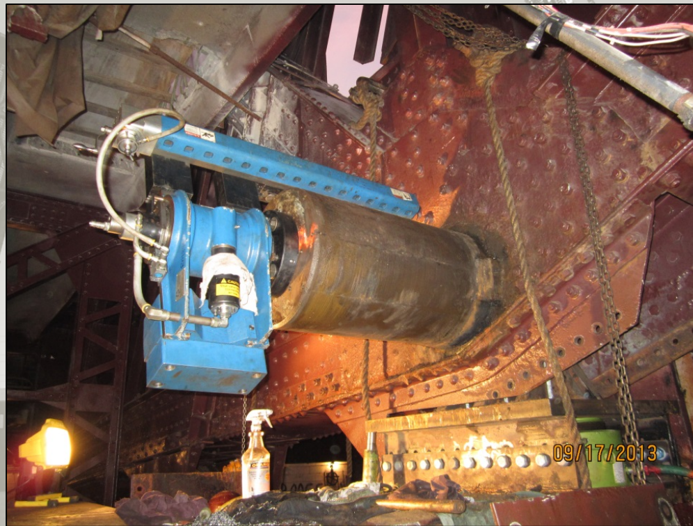
Field machining – Machine set up and aligned
