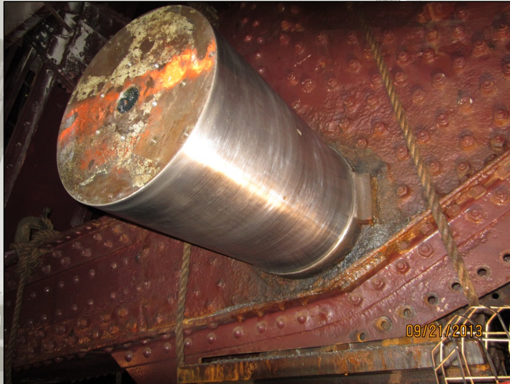
Field machining – Trunnion journal complete
