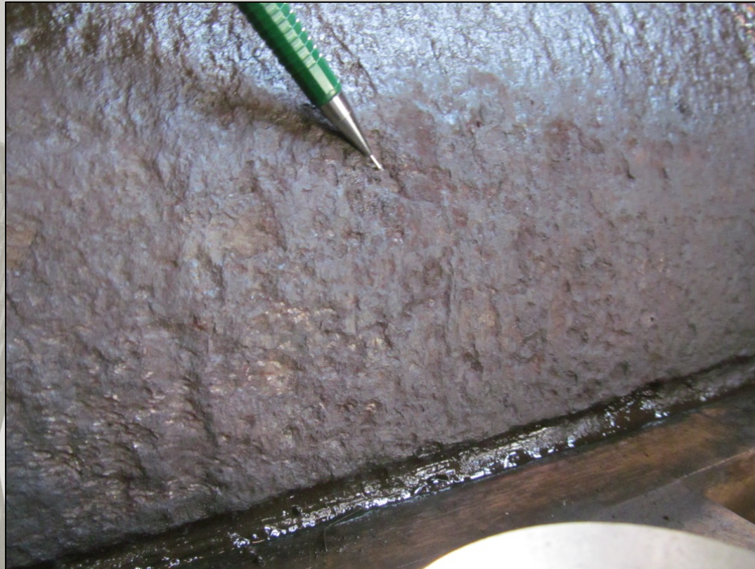
Outboard trunnion journal – close up of pitting
