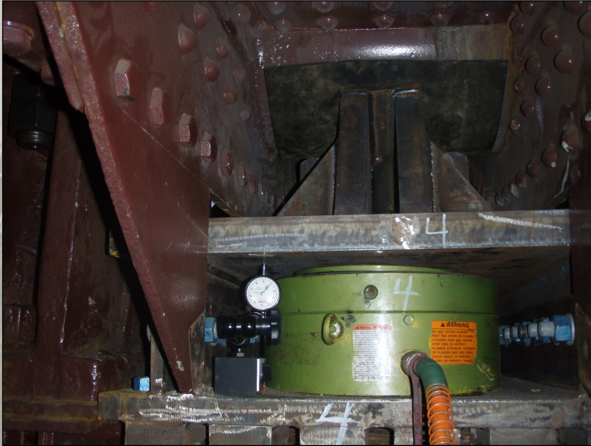
Up-close view of jacking saddle with jack
