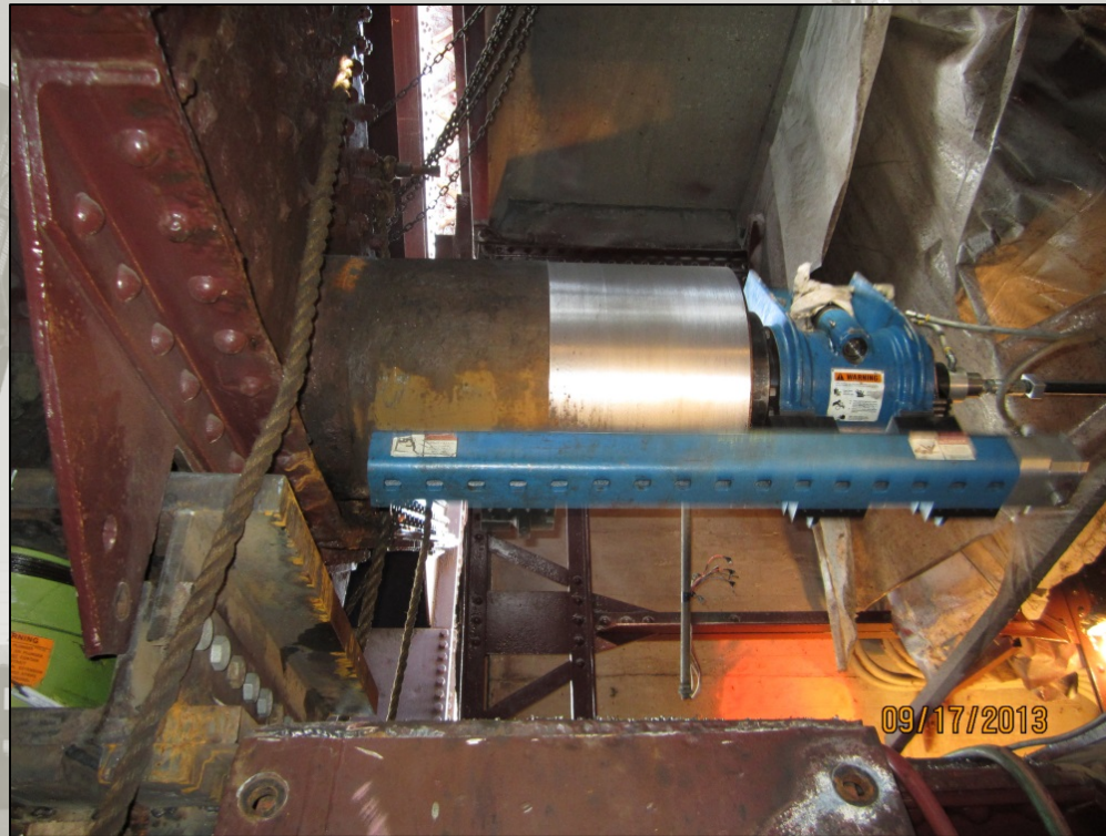
Field machining- Initial cut
