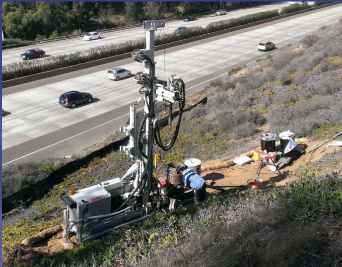
Drill rig (Pacific Drilling) at Arch Abutment 3
