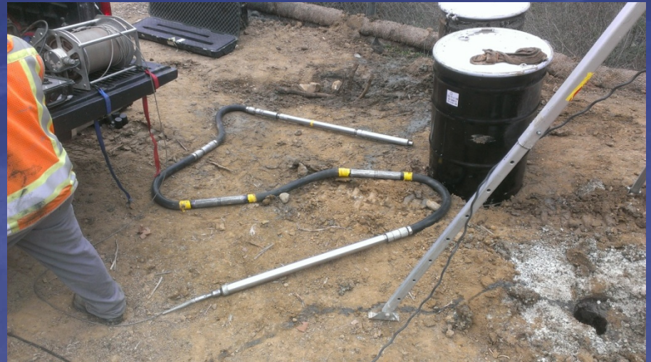
Downhole logging at Arch Abutment 2
