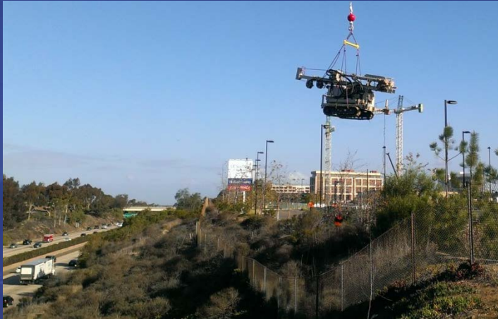
Craning in the drill rig at Arch Abutment 3
