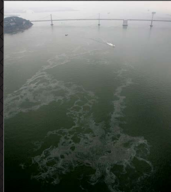
Ship Collision with San Francisco – Oakland Bay Bridge Main Pier Fender System
