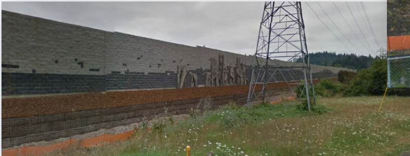
SB Ramp Soundwall
