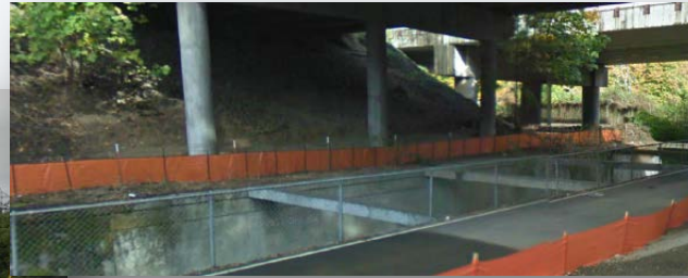
Canoe Canal Liner
