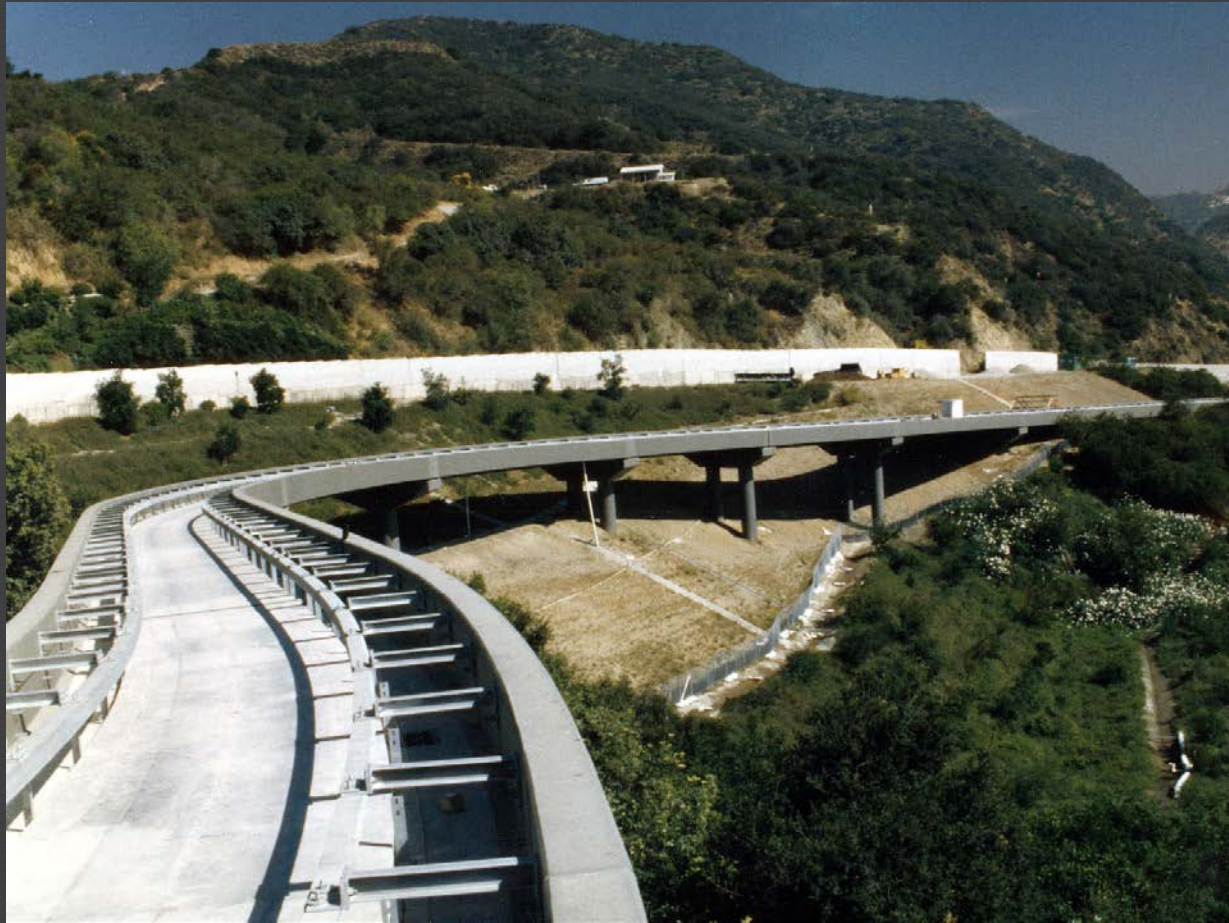
Guide rails secured to precast web elements
