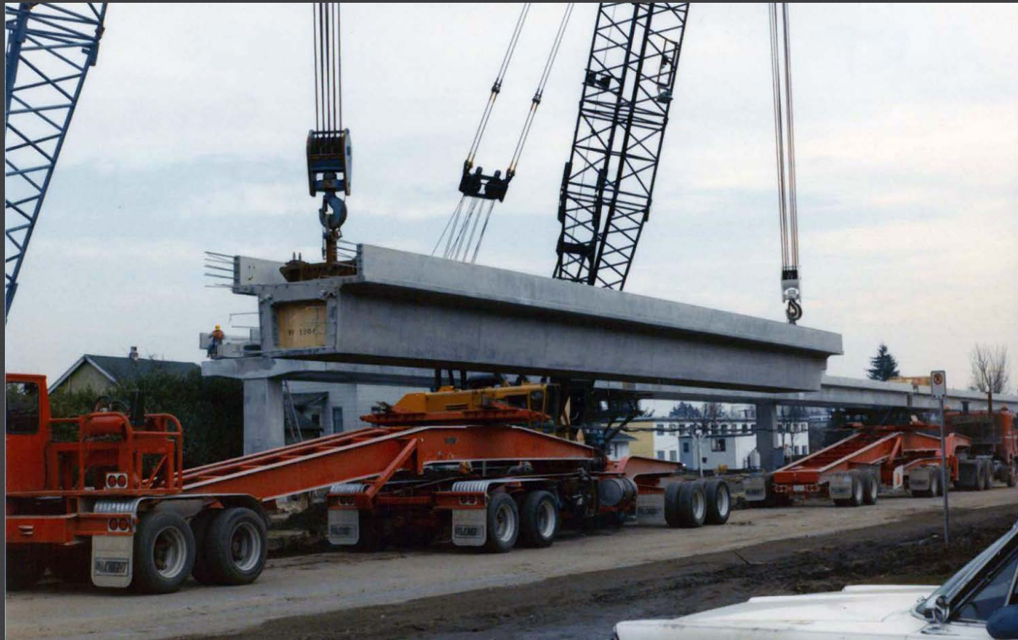
Typical 30m Guideway Beam
