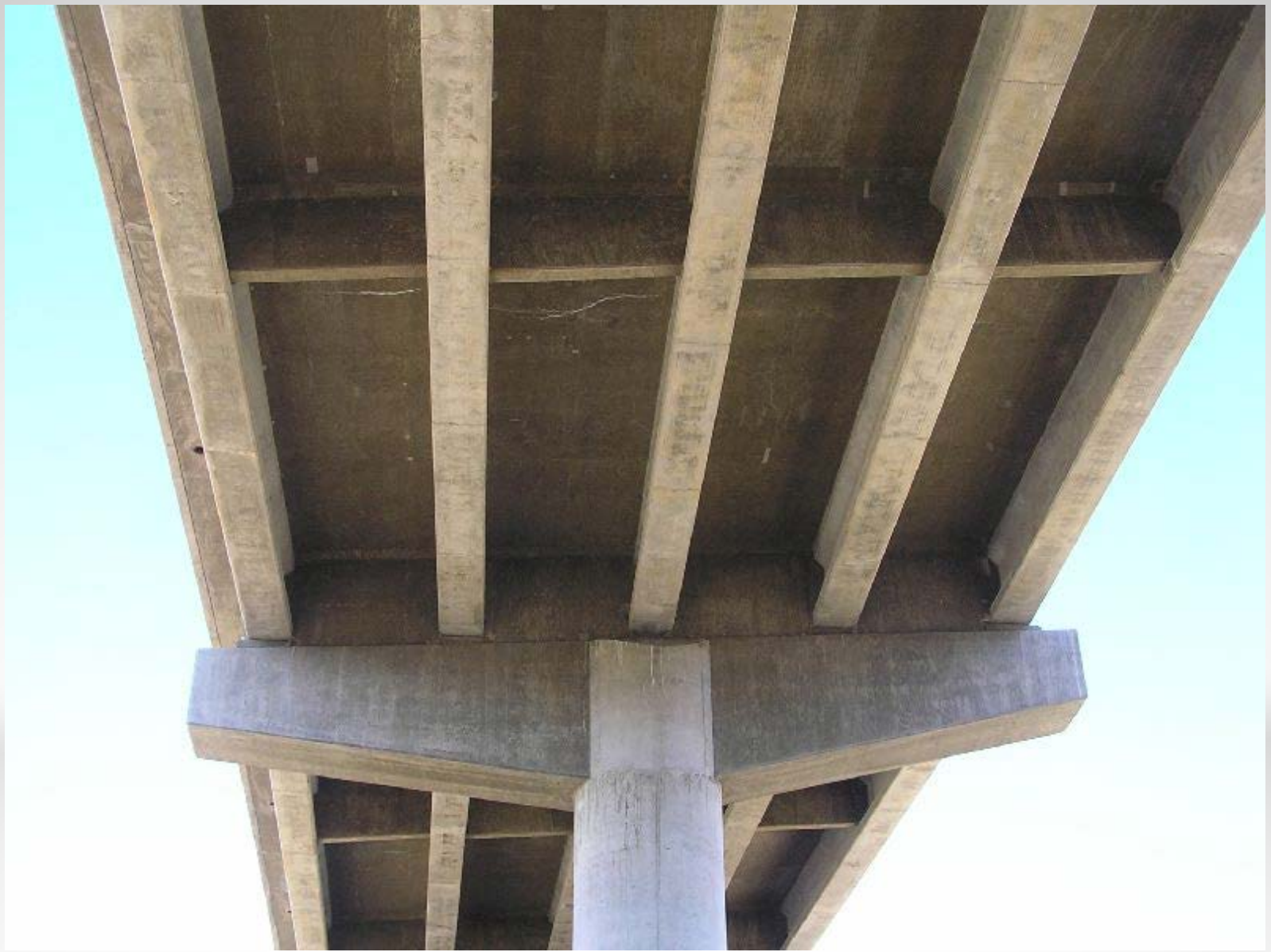
▶ Northbound Bridge Underside of Structure
