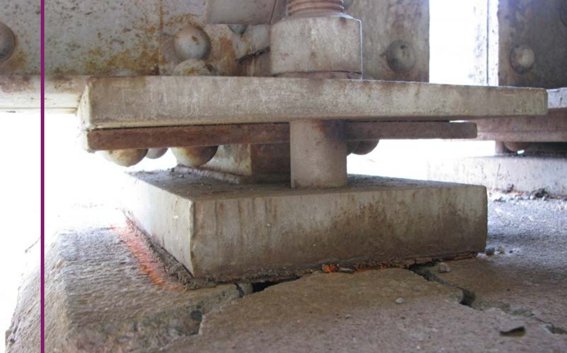
NE Bearing at Pier #3
