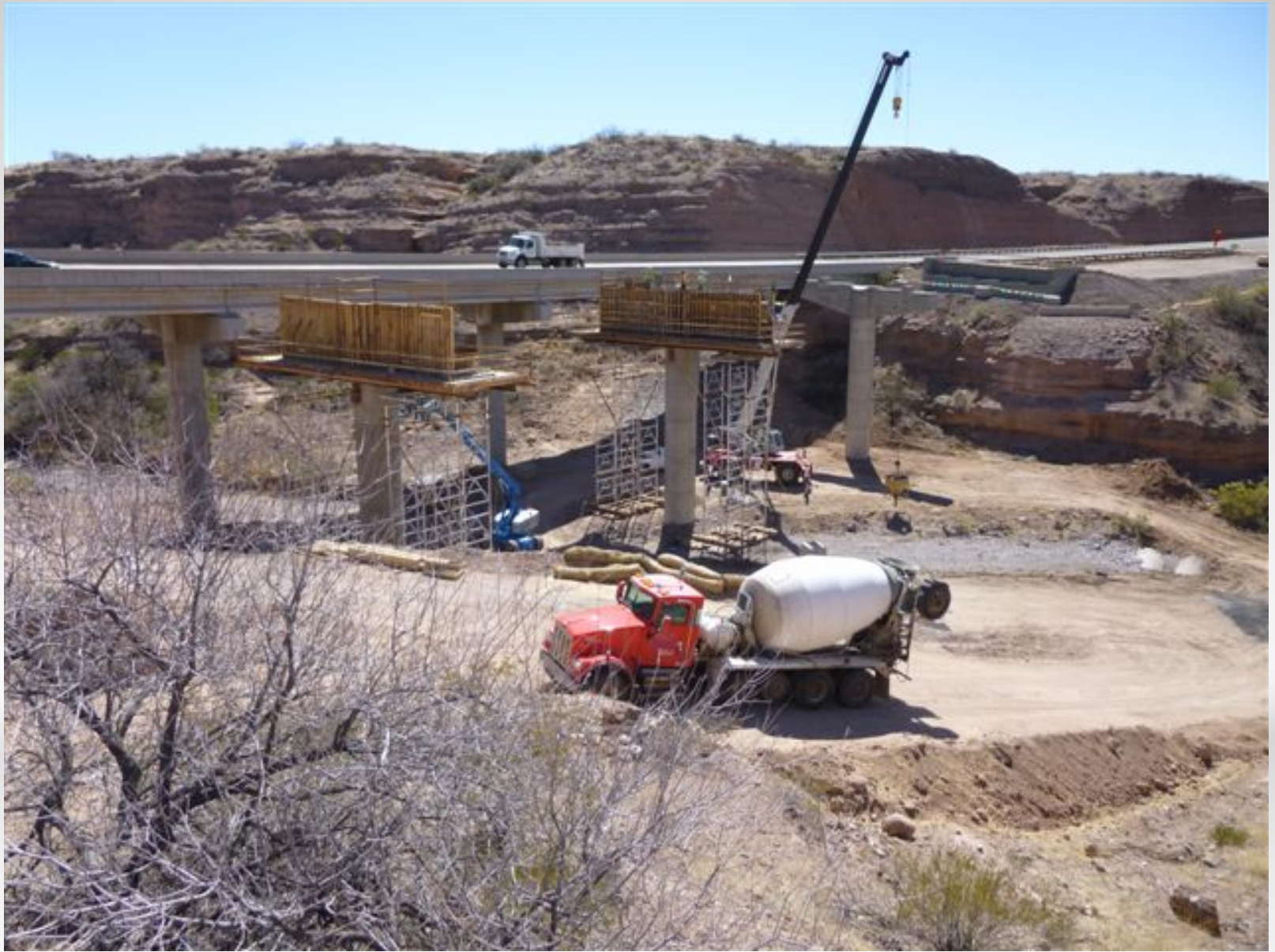
▶ Construction Access Road.
