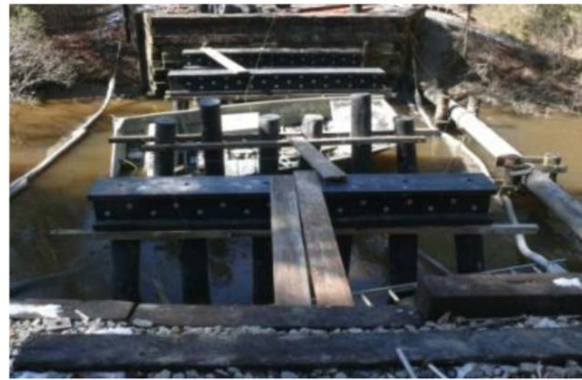
Pile Cap Installation
