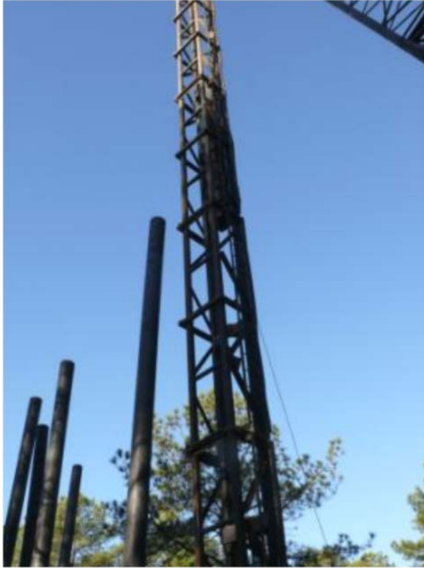
Driving RSPC Piles
