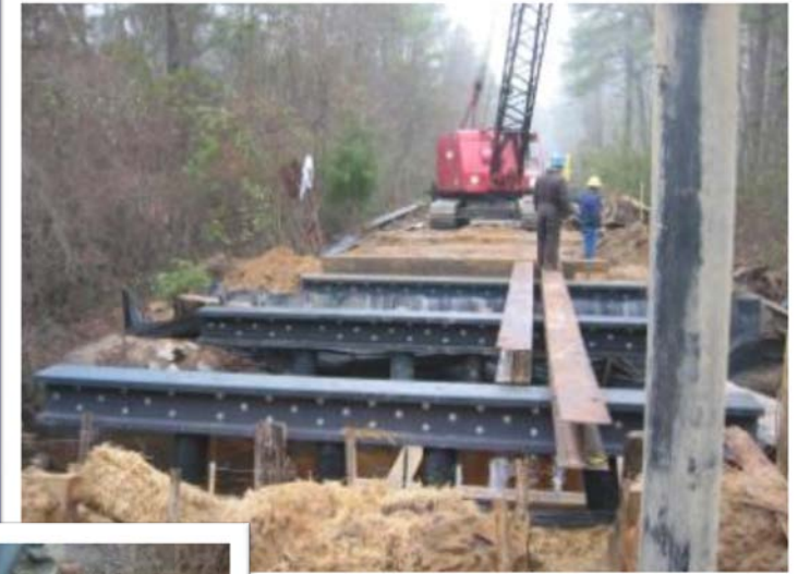
Pile Cap Installation
