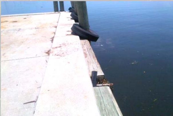
Pier Fenders & Pilings
