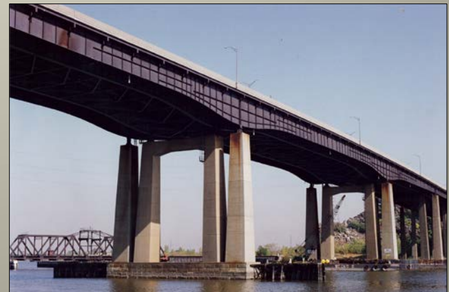
Continuous River Spans Unit
