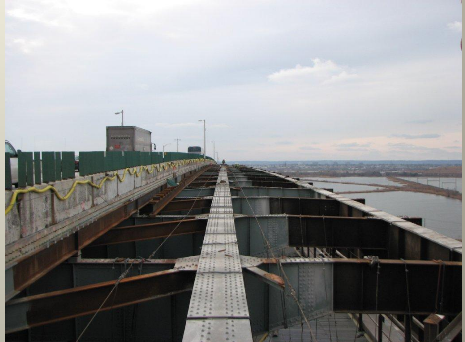
Girders and Floorbeams Stripped of Stringers
