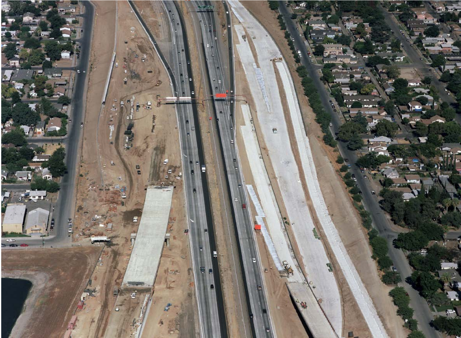
Aerial View- July 2013
