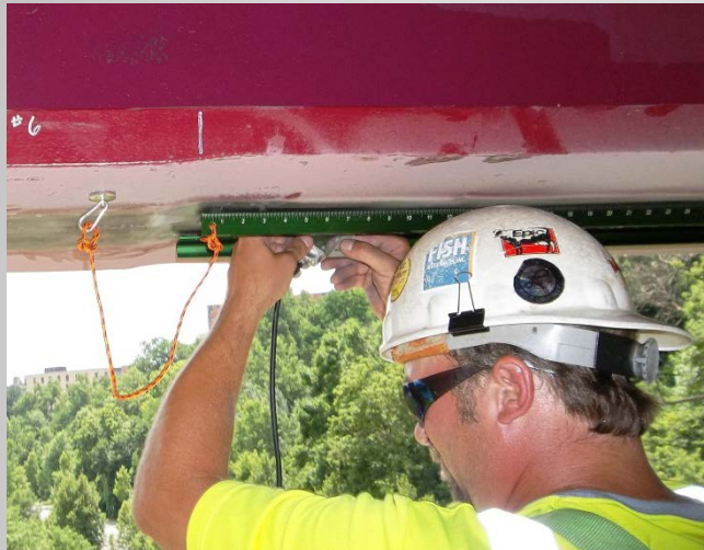
Scanning parallel with weld axis
