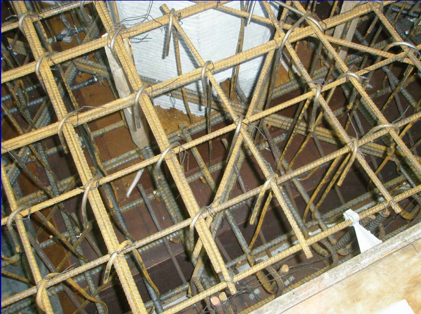
Diagonal “shear friction” steel. Vertical stirrups.
