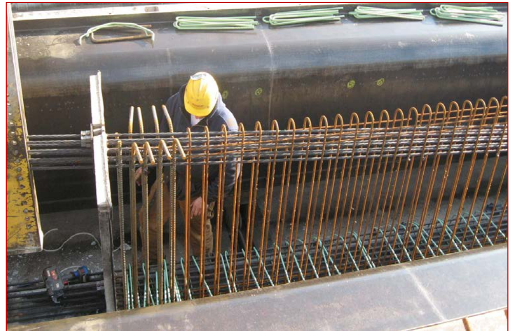
Steel reinforcing bars
