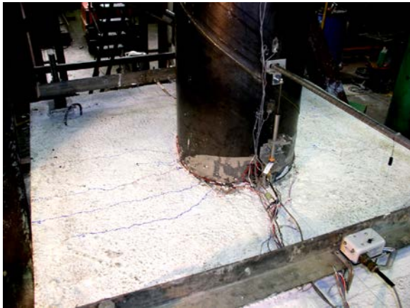
limited footing damage: 2.5% drift
