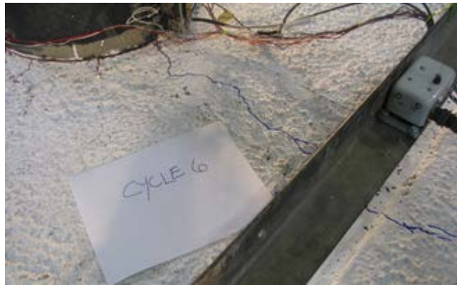
bisecting cracks: 0.75% drift
