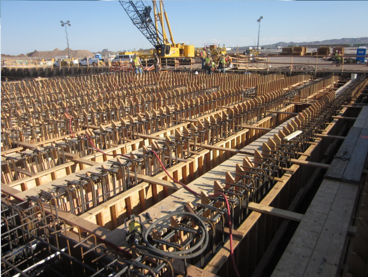
SEPT. 2012: FORMING BOTTOM SLAB AND WEBS
