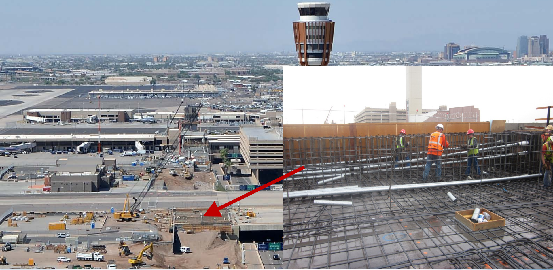
SEPT. 2012: FORMING BOTTOM SLAB AND WEBS
