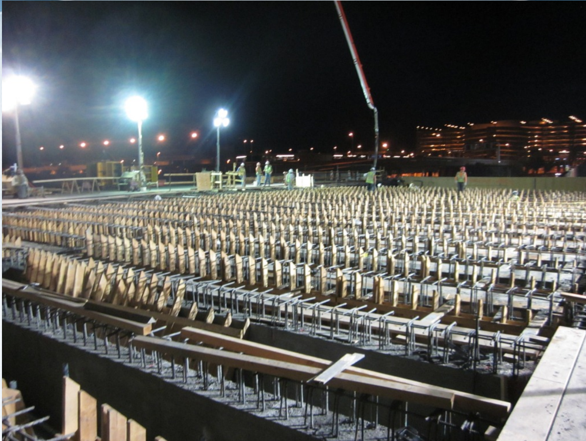
SEPT. 2012: POURING BOTTOM SLAB AND WEBS
