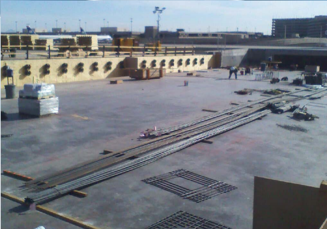
AUG. 2012: WASTE SLAB CAST AGAINST SOFFIT FILL
