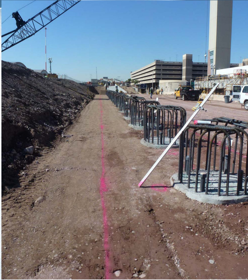
JUNE 2012: INSTALL ABUT. 1 DRILLED SHAFTS
