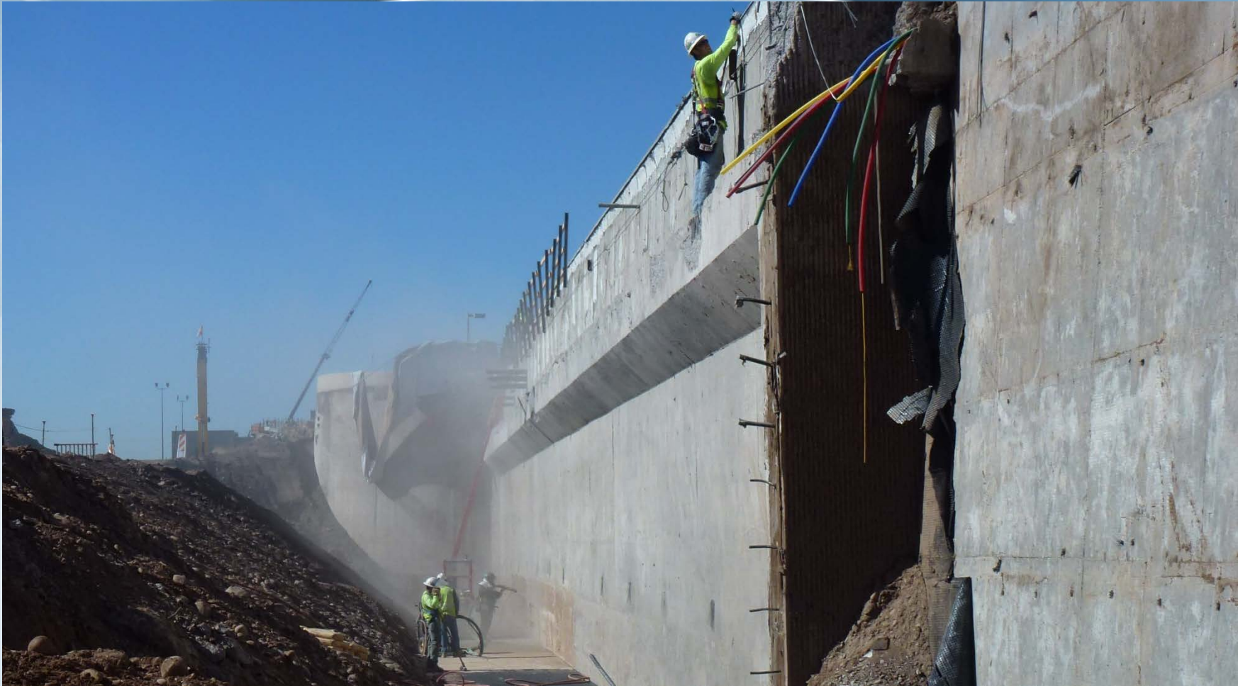
MAY 2012: PREP. EXISTING ABUTMENT SURFACE
