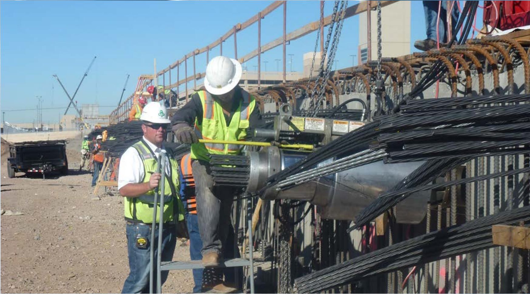
OCT. 2012: POST-TENSIONING
