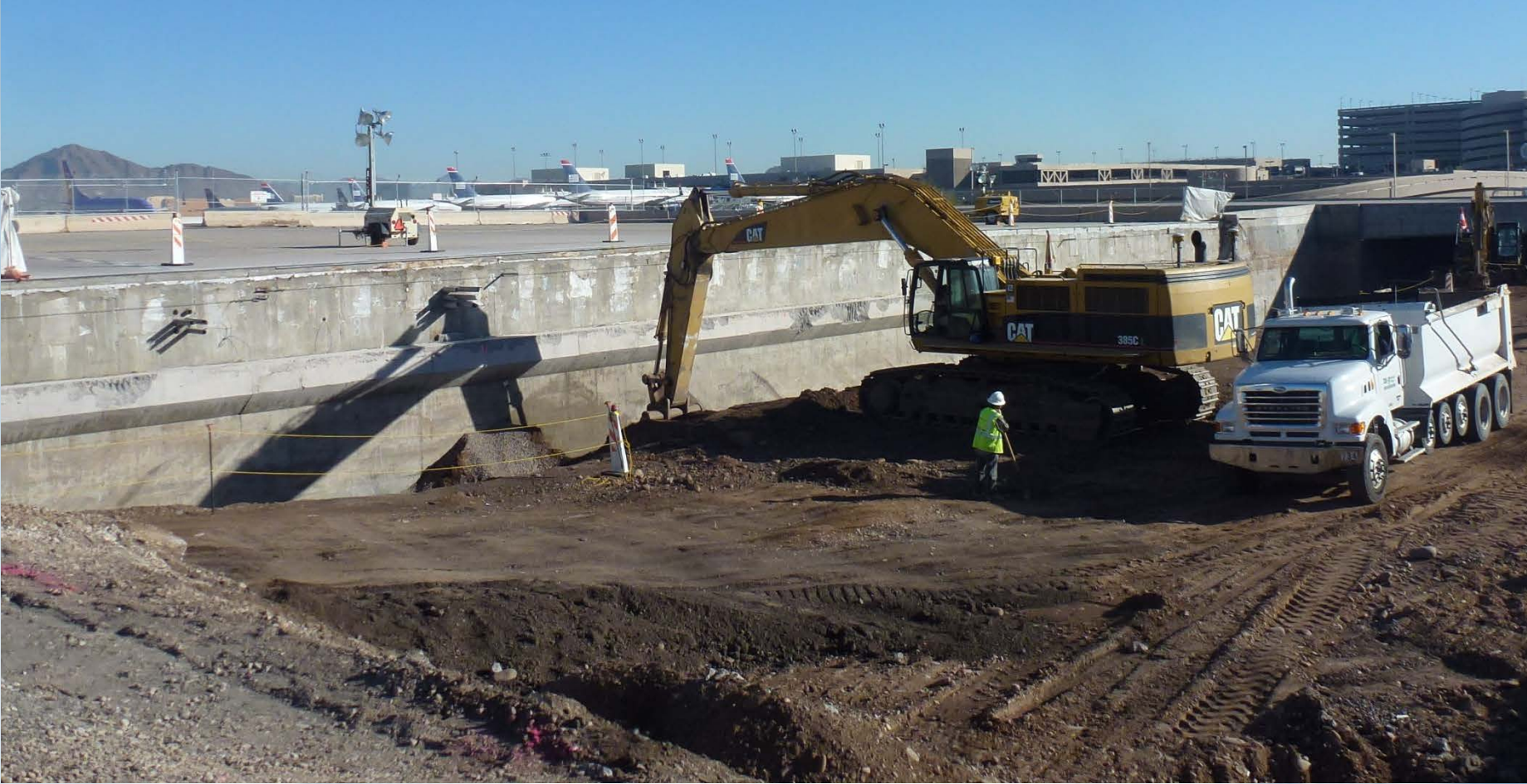
MAY 2012: EXCAVATE ADJACENT TO EXISTING ABUTMENT
