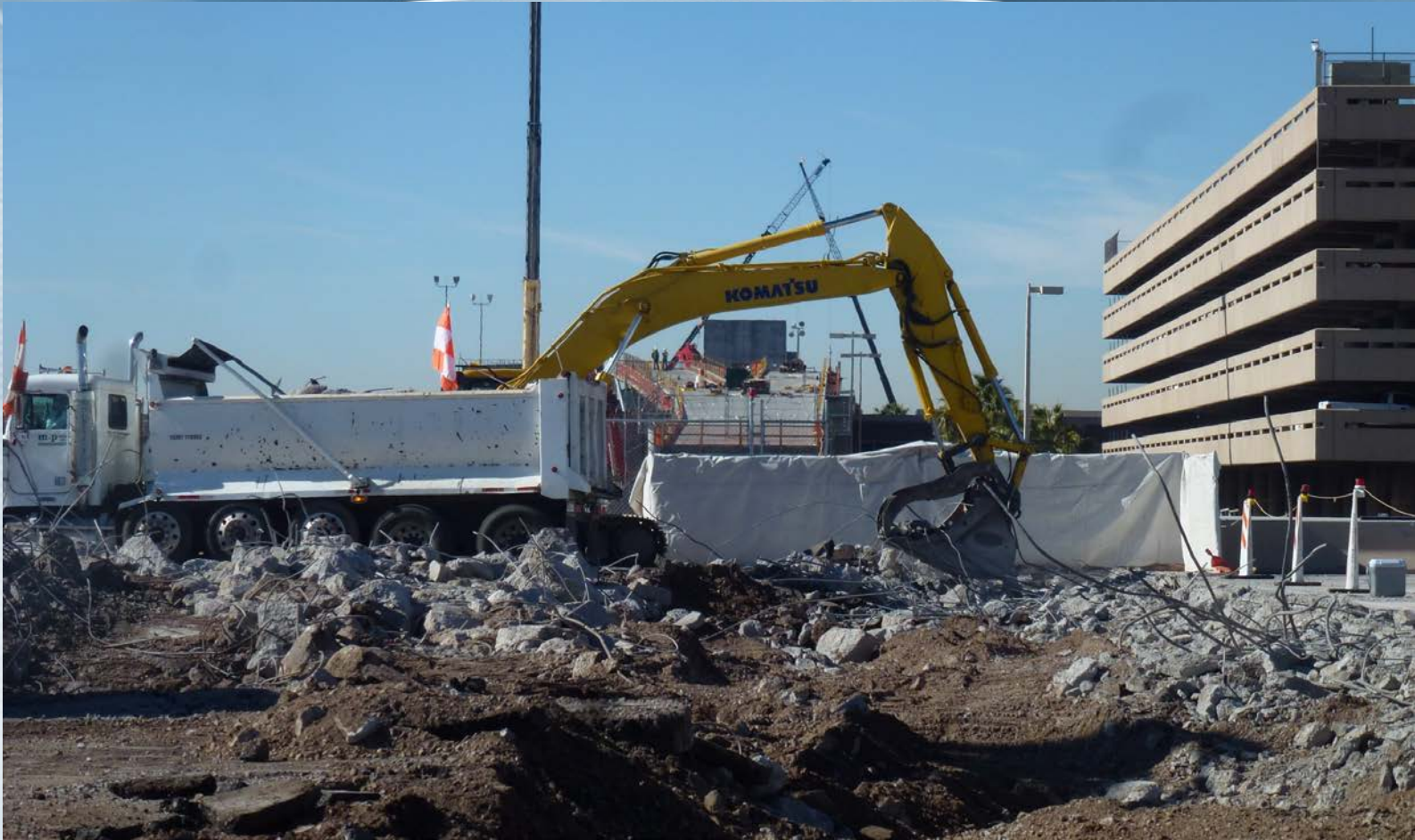
MAY 2012: DEMO EXISTING TAXIWAY 'S'
