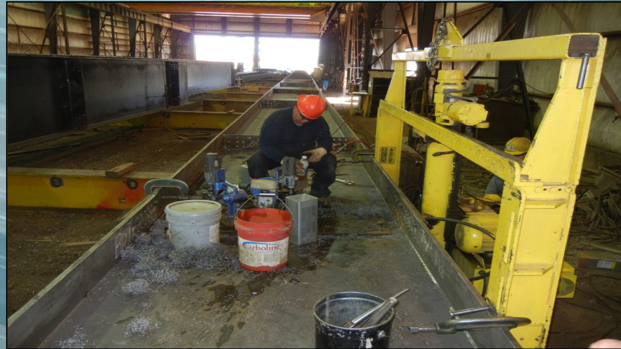
Drilling Holes in Web for Field Splice Connection
