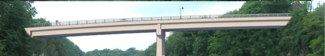
Prestressed Concrete Girder
