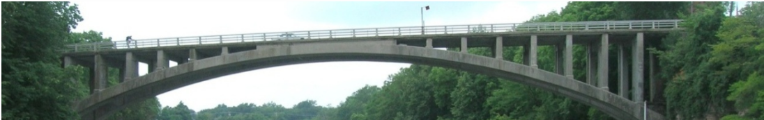
Existing Concrete Deck Arch
