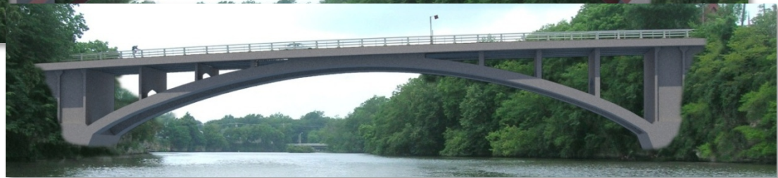
Concrete Deck Arch
