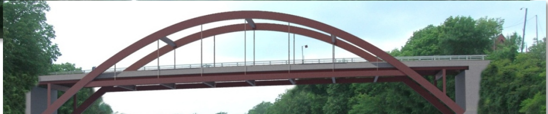
Partial Thru Steel Arch
