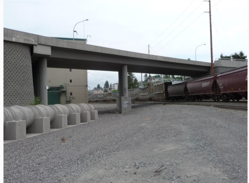
Elevation View Looking North
