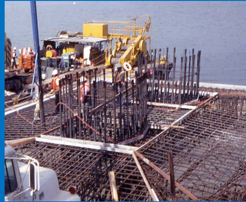
Column main bar couplers at the base
