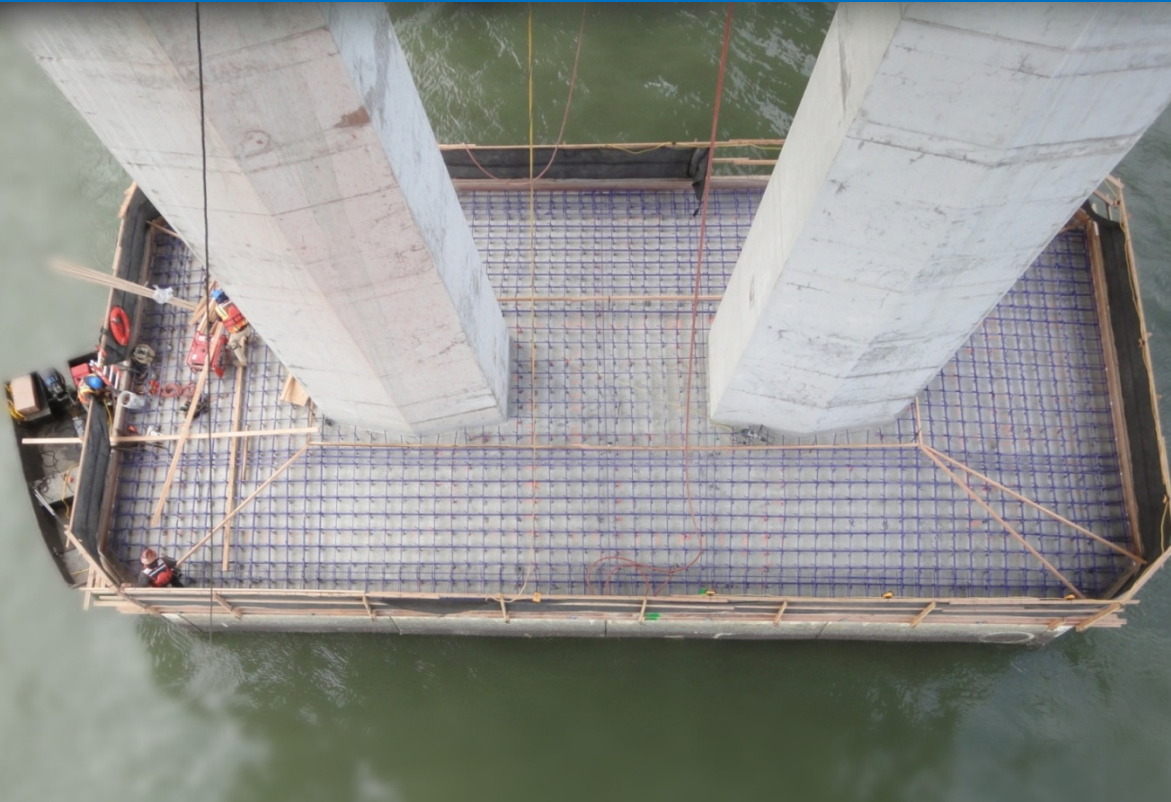
Footing pile cap strengthening
