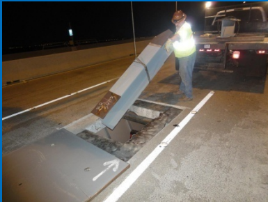
Deck Opening for Hauling Material
