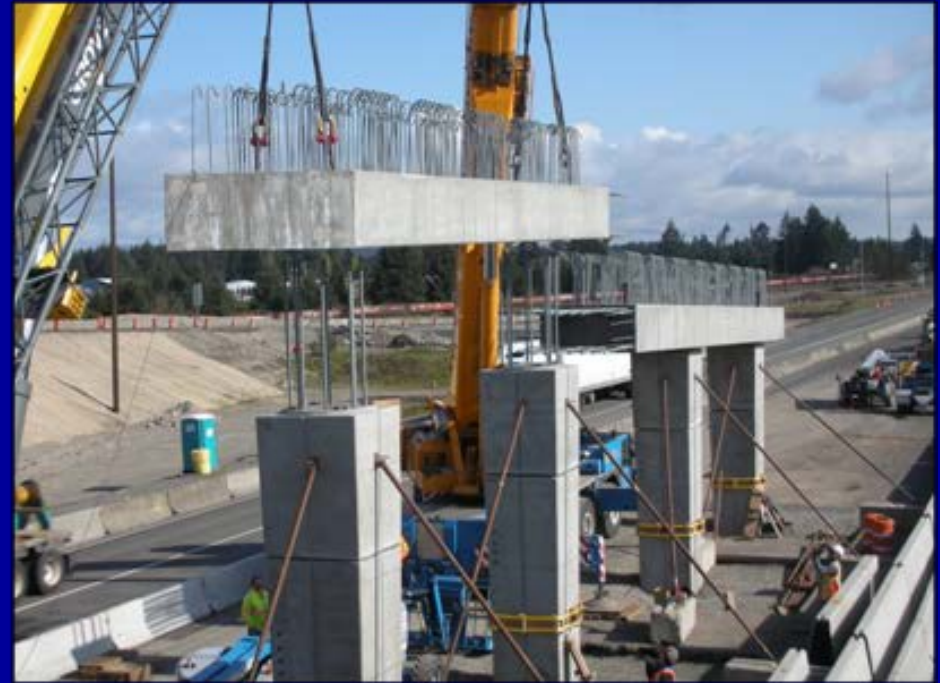
Cap-Beam Connection
