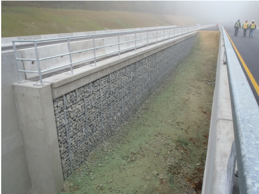
Wire-faced MSE median wall
