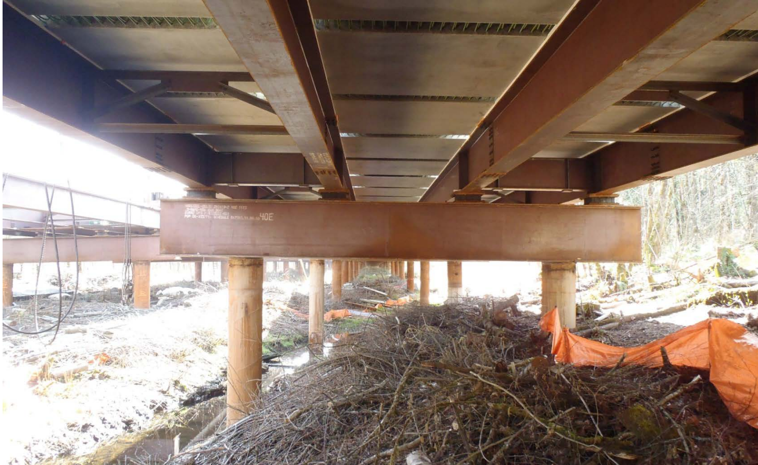
Piles, caps, girders, precast deck panels installed
