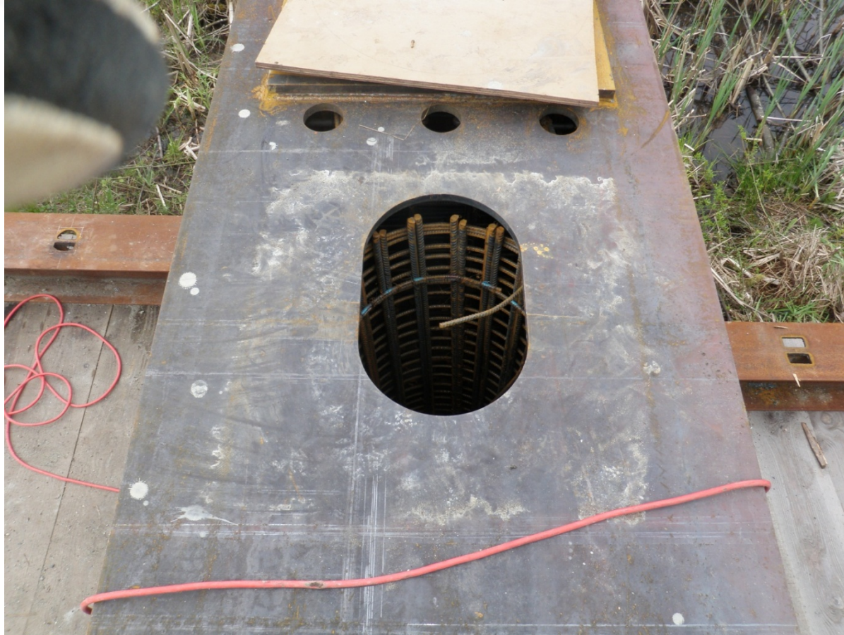
Pile rebar cage projects into pilecap joint
