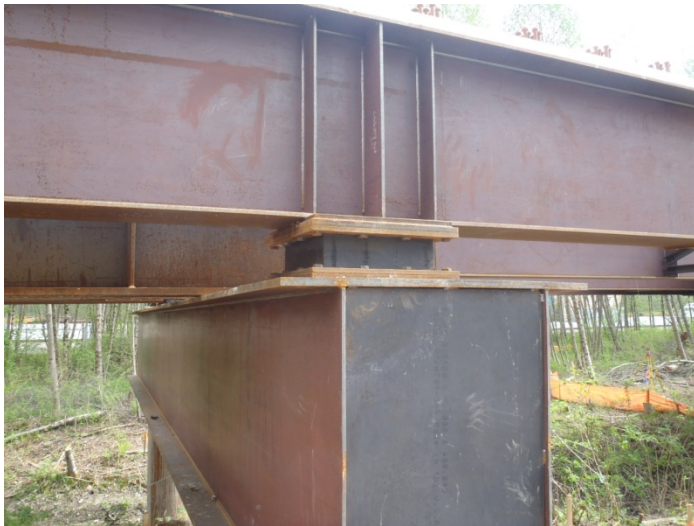
Typical single-bearing support
