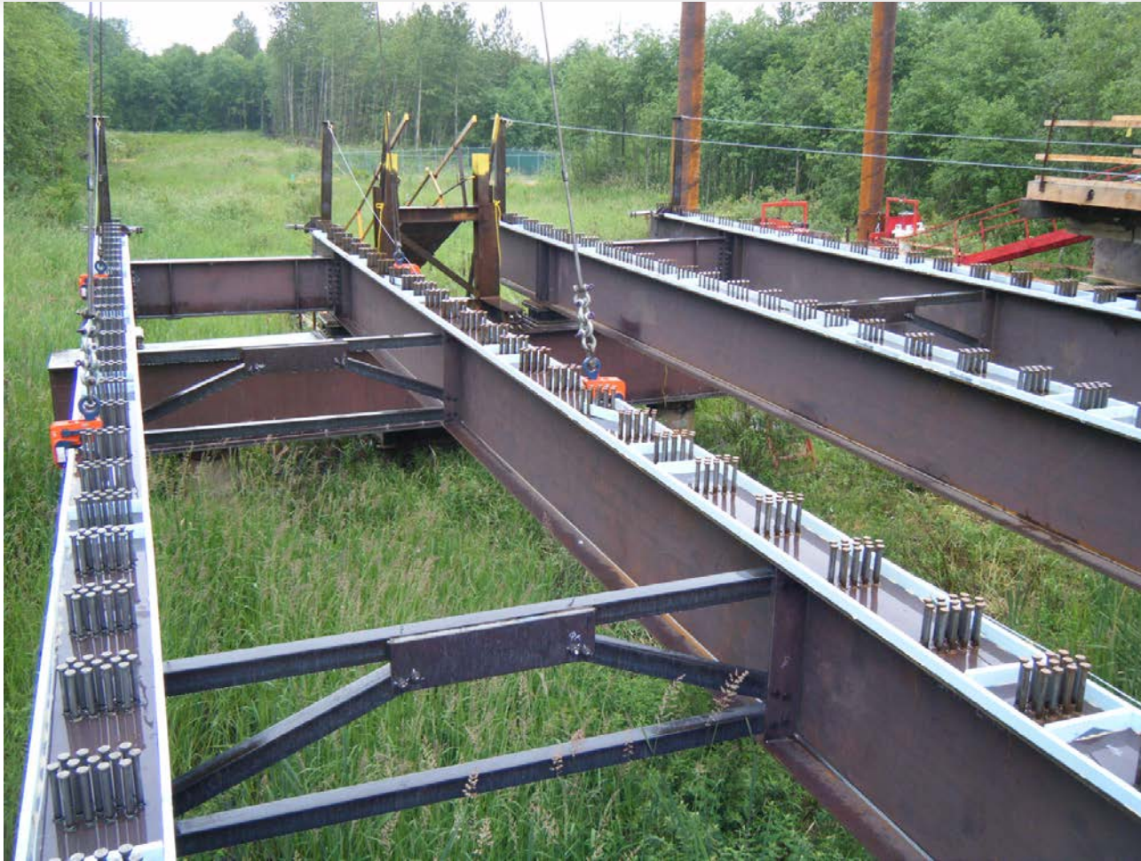
Girders lifted in braced pairs
