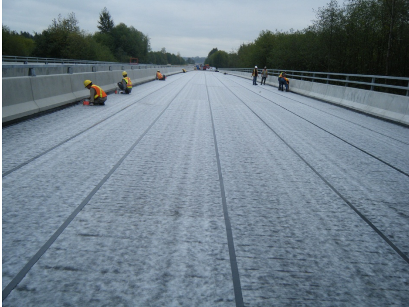
Installation of Protecto Wrap preformed waterproof membrane
