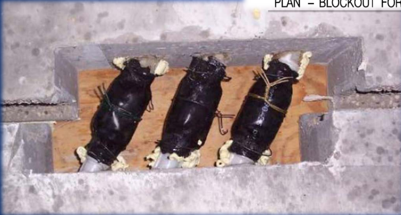
PLAN - BLOCKOUT FOR POST-TENSIONING DUCT
