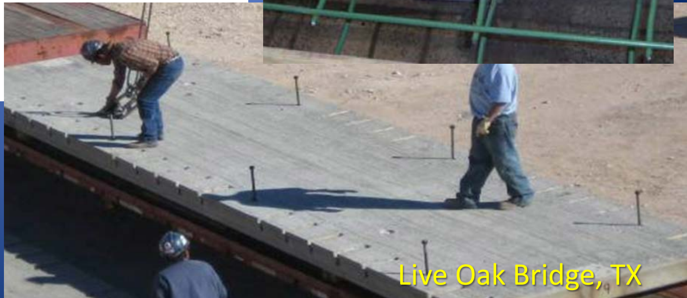
TYPICAL SECTION LEVELING DEVICE
