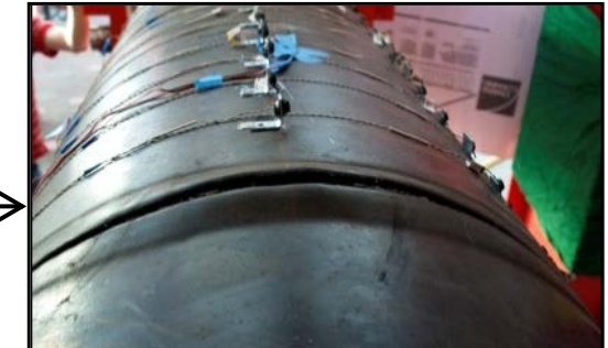
Rupture at Ductility 6 pull 2
